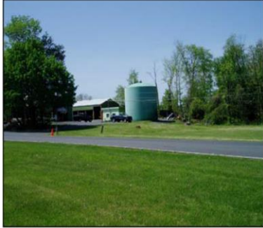
Water storage tank.
