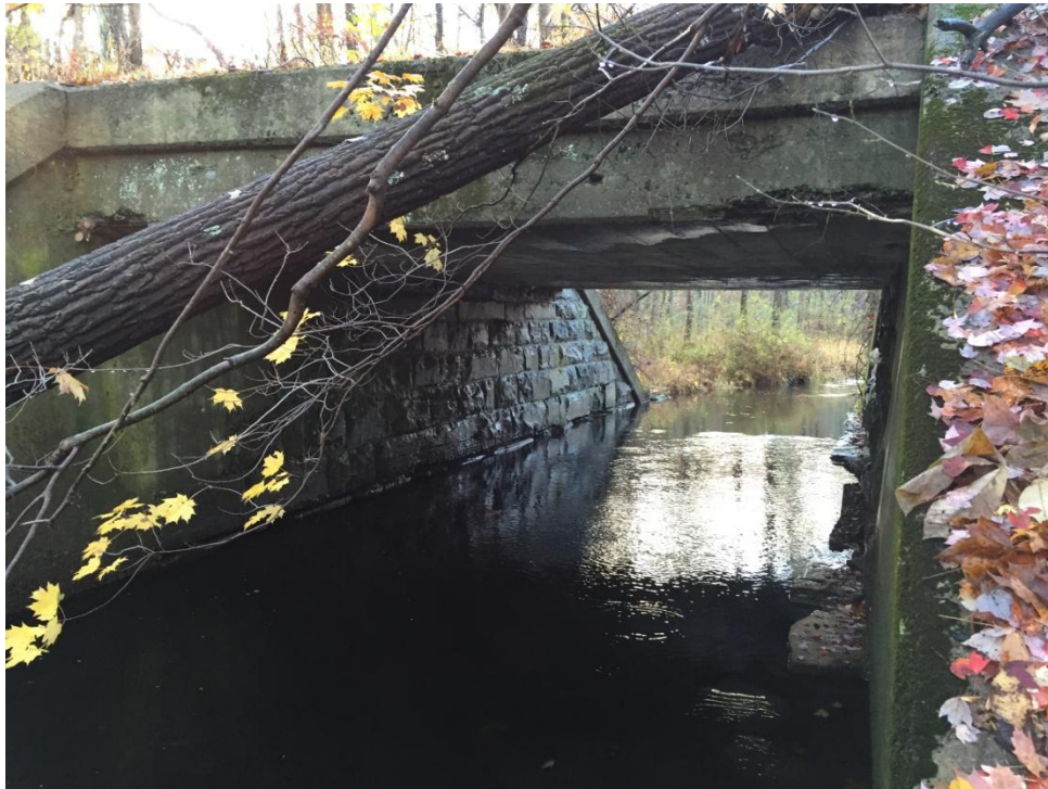
Photo 8 - This picture was taken looking south at the existing culvert crossing the Black Creek.
