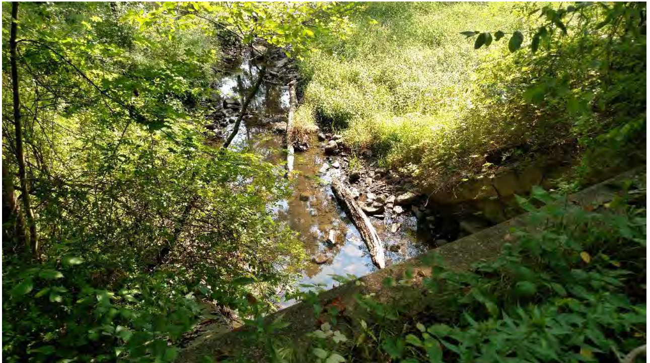
Photo 16: In some areas, the project corridor is significantly raised above grade: in this photo approximately 10'. View to the south.
