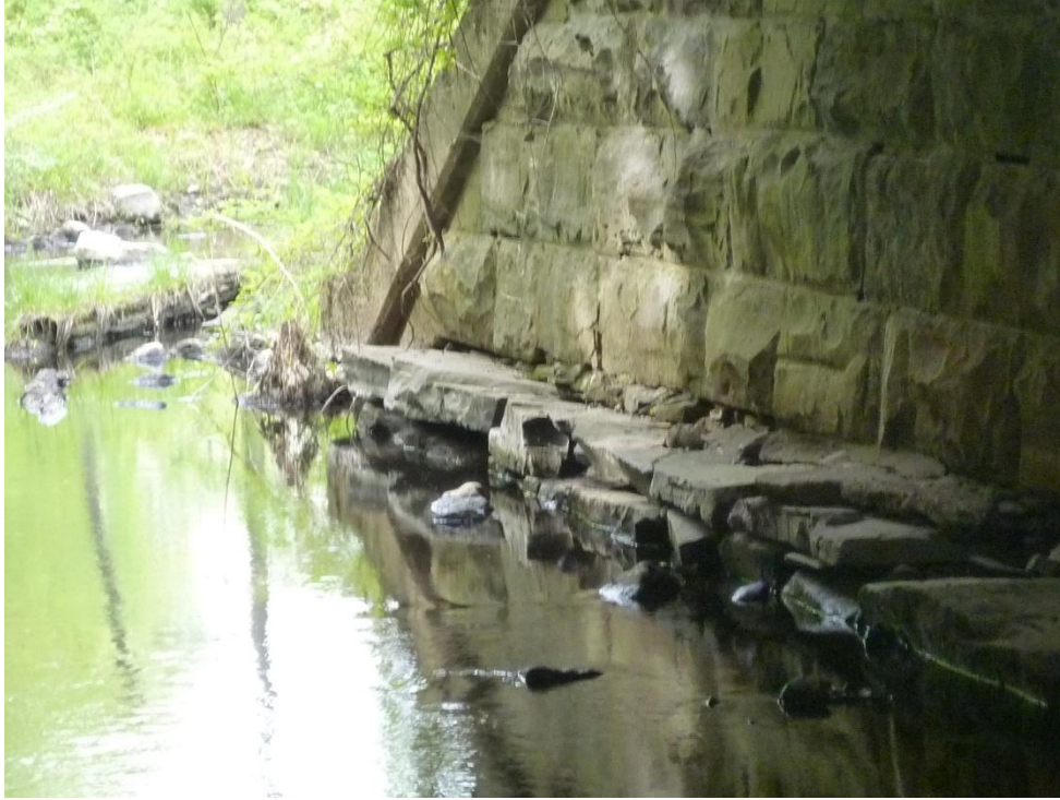
Photo 7- This picture shows the general condition of the existing abutments/wingwalls of the culvert crossing the Black Creek.
