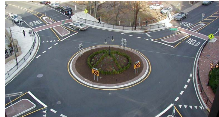
Gateway roundabout in Town of Great Neck Plaza, NY
