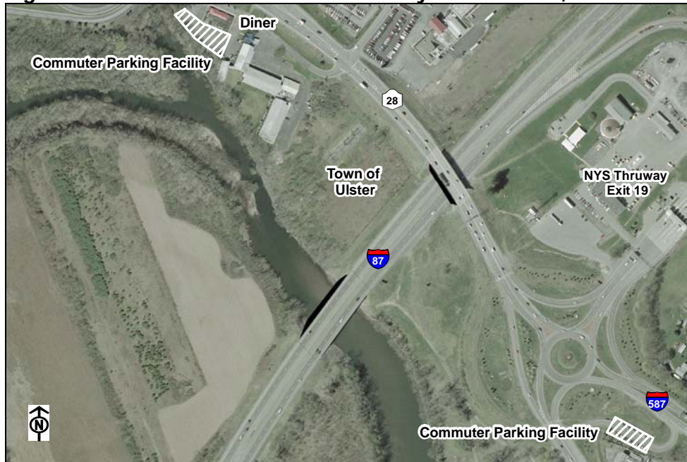
Figure 3: SR 28 at I-587 at NYS Thruway Exit 19 Area, Town of Ulster
