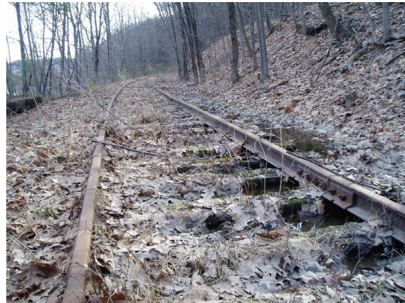
Railroad side slope bench locations force RWT to cut into the slope or fill the outside. Either option will cause clearing and drainage problems, likely require retaining walls and cause dramatic escalation in costs.
