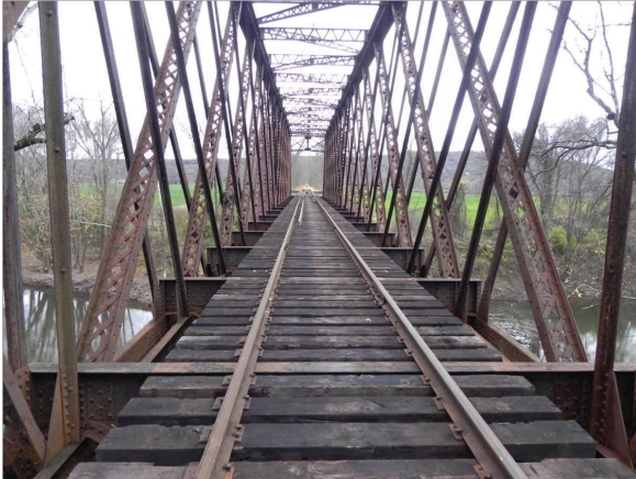
At the C-9 bridge over the Esopus RWT would require extending the trail outside the superstructure or hanging the trail below the bridge.
