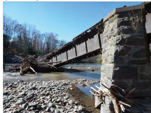
Although east of Phoenicia the Boiceville Trestle was destroyed by Irene and separates the rail from the Ashokan Reservoir
