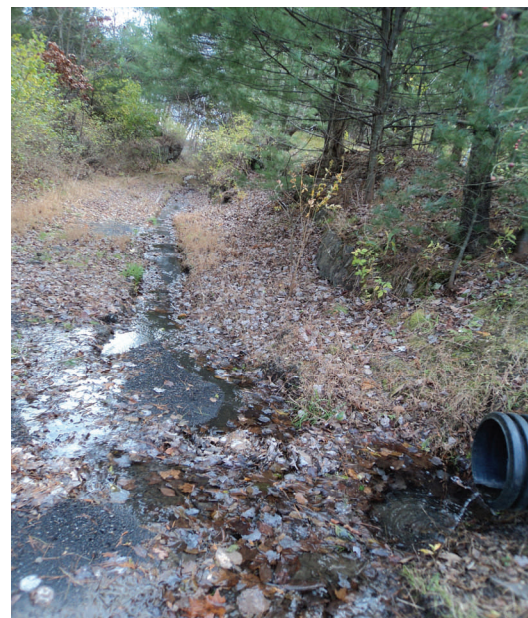
RWT would require greater investment to address drainage issues including culverts and swales.
