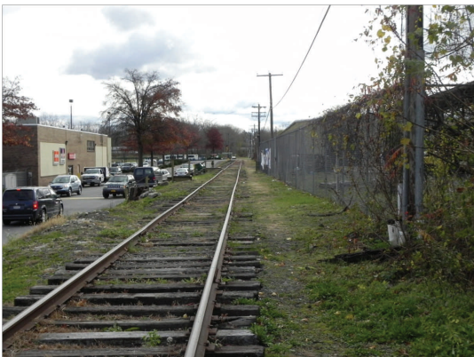
At Kingston Plaza RWT would require either relocation of business activities and utility poles or encroachment into travel lanes .
