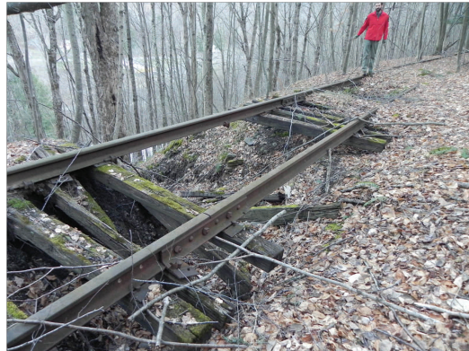
Washout near Pine Hill
