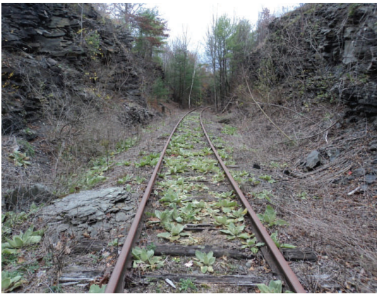
RWT would require either removal of rock to run along side the rail in the cut or find a way both up and down to run along the top of the cut.
