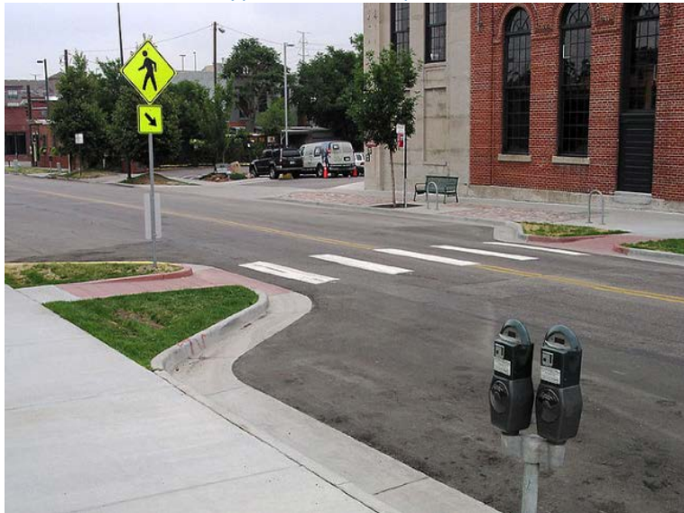
Typical Curb Bump Out
