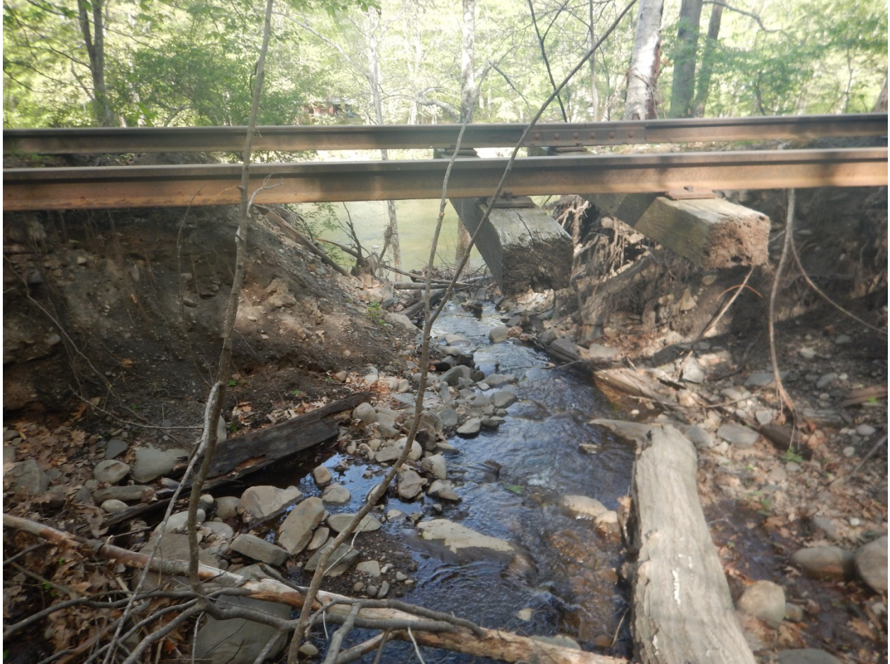
Example of a washout which may have been caused by a blocked culvert. Allowing debris to build up around culverts can cause the drainage path to be redirected, causing the roadbed and ballast section to be washed out.
