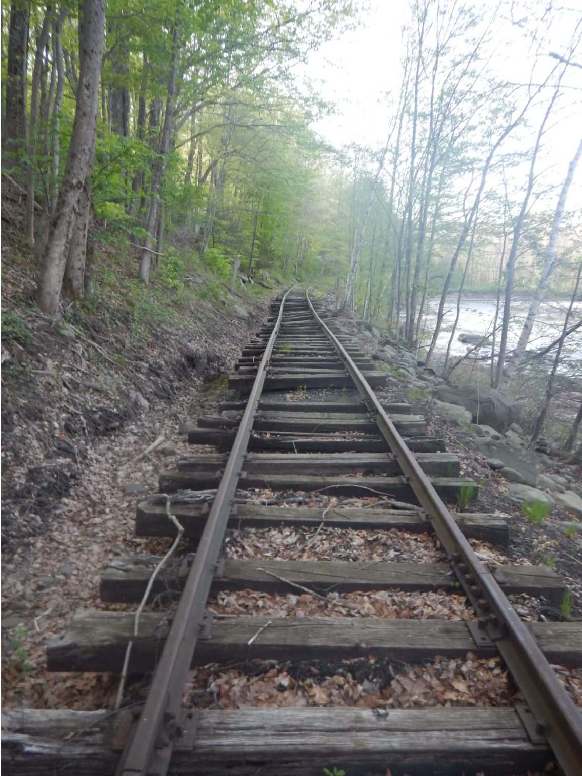
Example of a washout caused by a ditch becoming flooded from heavy rainfall. Stormwater that could not flow naturally to a culvert would flow laterally over the track structure, washing away ballast. The final result of this would leave the track in inoperable condition.
