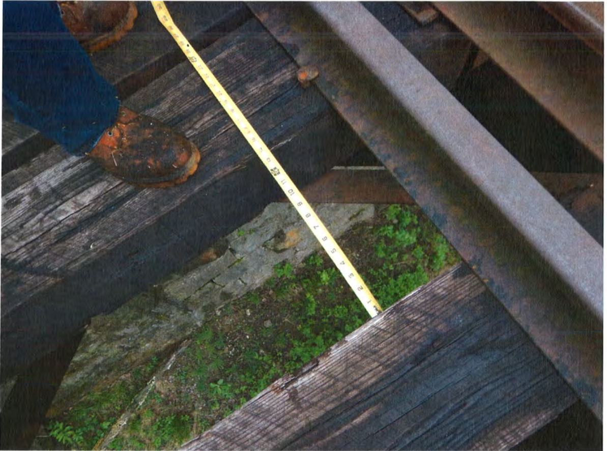
Photograph showing longitudinal shifting of a bridge timber, creating a condition where a person could fall through.
