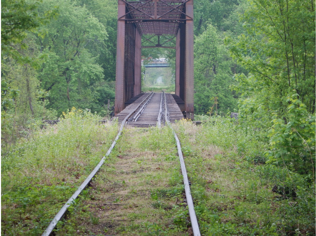
Eastward photograph showing alignment deviations on both approaches of the C9 Bridge. HDR advised the County to cease operations over this bridge until the structure can be evaluated. HDR Track Inspectors observed that the concrete abutments have shifted.
