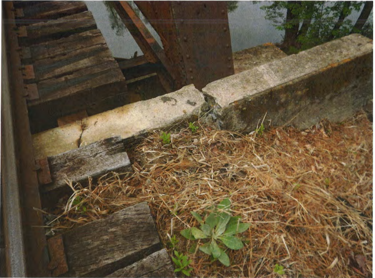
Photograph showing the eastern bridge abutment. The movement has allowed the roadbed to destabilize which is non-compliant with FRA Rule 213.103(a).
