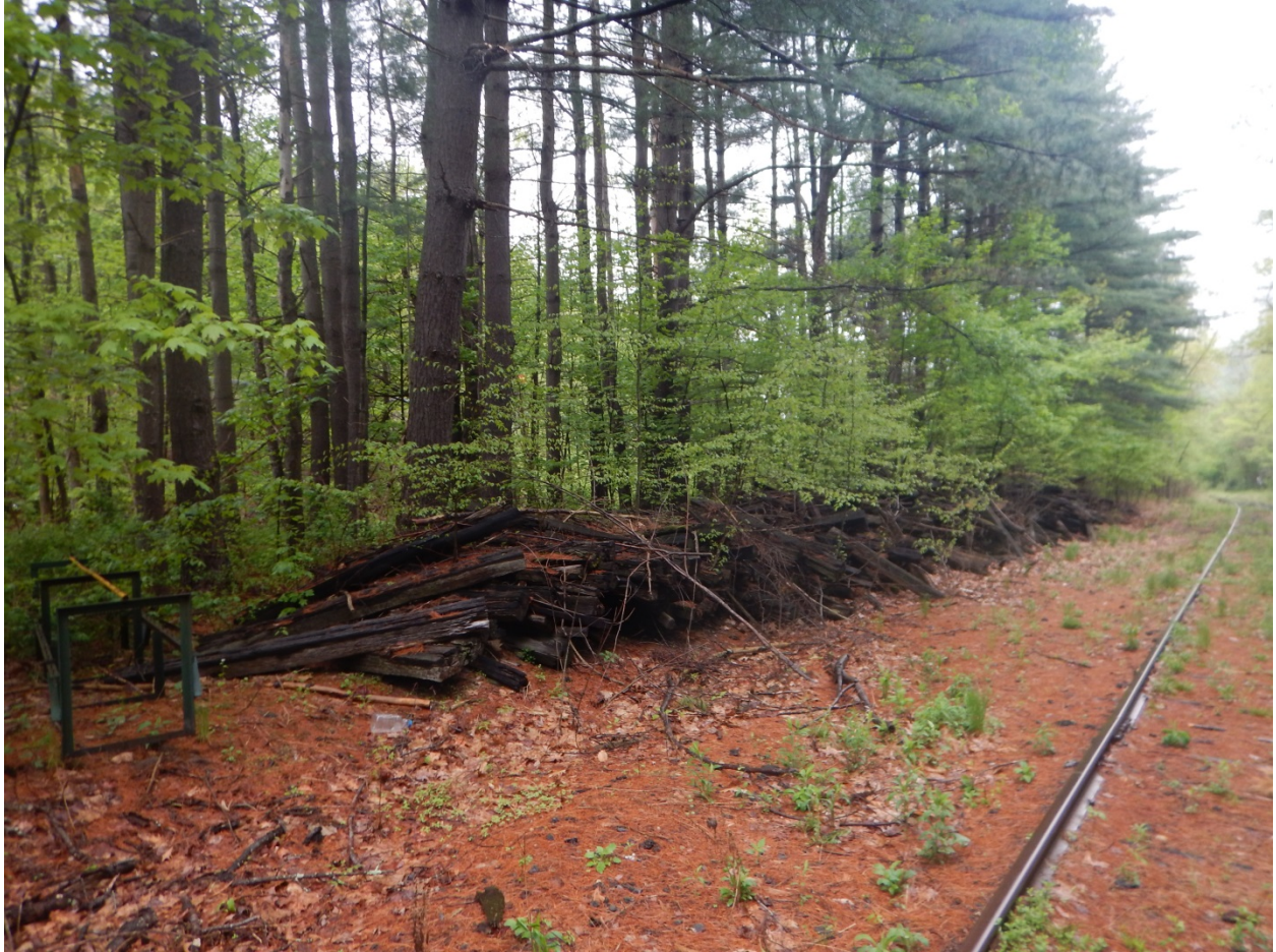
Example of tie piles left along the right of way. Ties should be disposed of at an approved facility.
