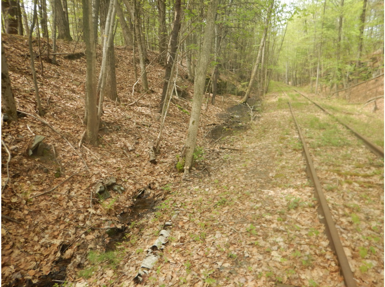
Example of a ditch where debris and sediment have accumulated over time. Note the trees that have grown in the area. Routine ditch maintenance ensures proper stormwater flow and prevents vegetation from growing and fouling the waterway.
