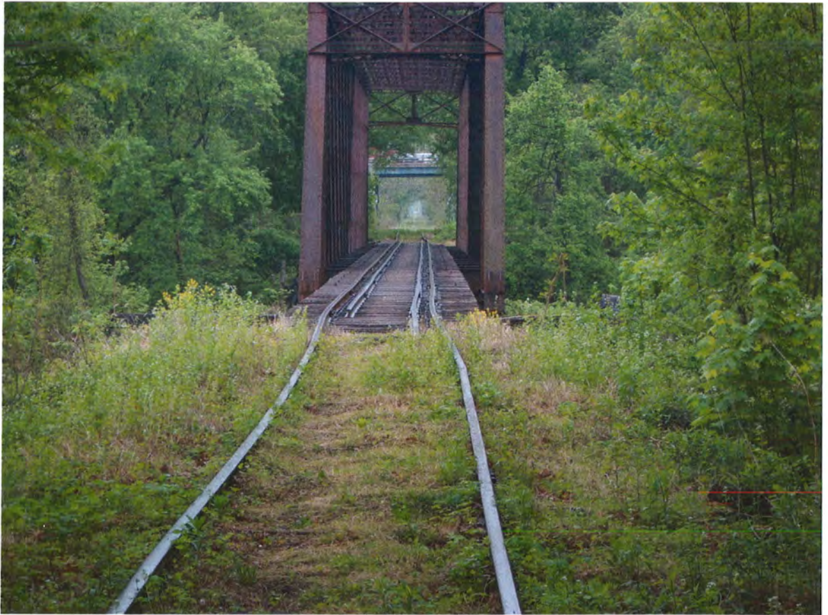
Eastward photograph showing the alignment deviations on both approaches.
