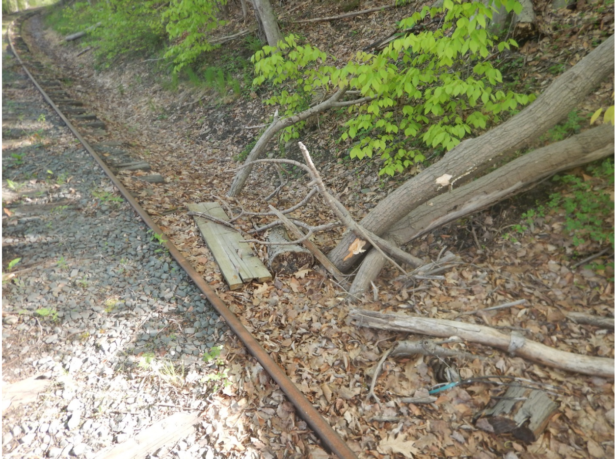
Example of debris accumulating in a ditch.
