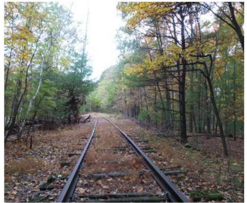
Photo 1-2 – Existing Rail Infrastructure Conditions – Segment 1
