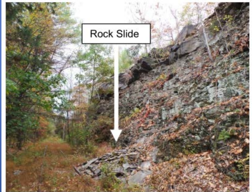
Photo 1-5 Rock Slide in Segment 1
