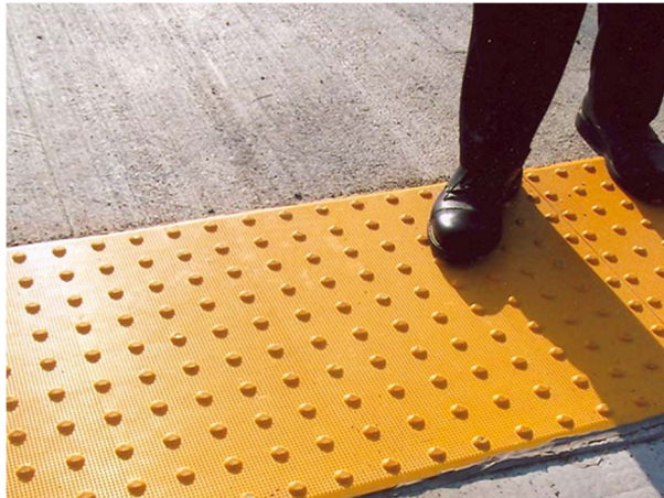
Truncated dome/tactile warning strip
