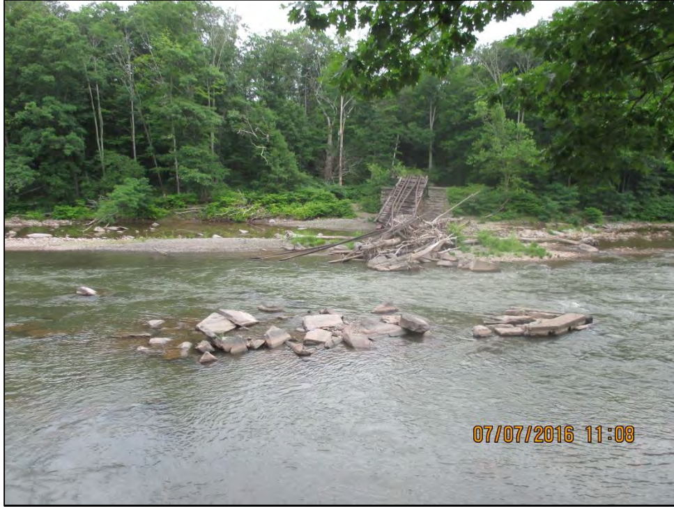
Photo 9. View looking west at proposed Espopus crossing. "Boiceville Trestle" destroyed by Tropical Storms Irene and Lee.
