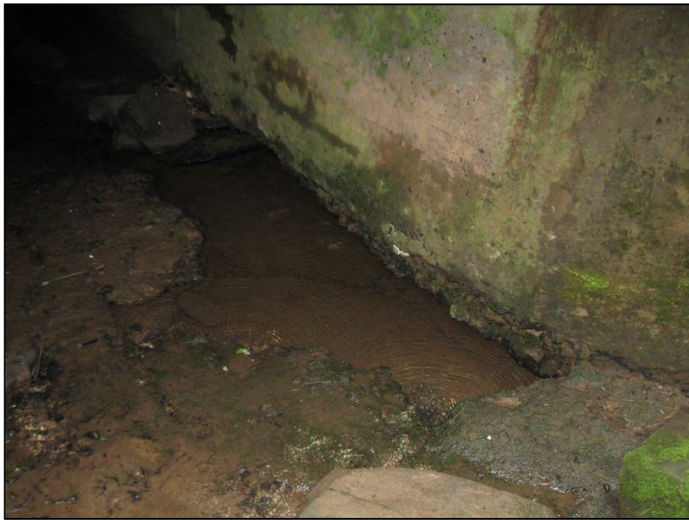
Photo 18. Flow of stream through large culvert.
