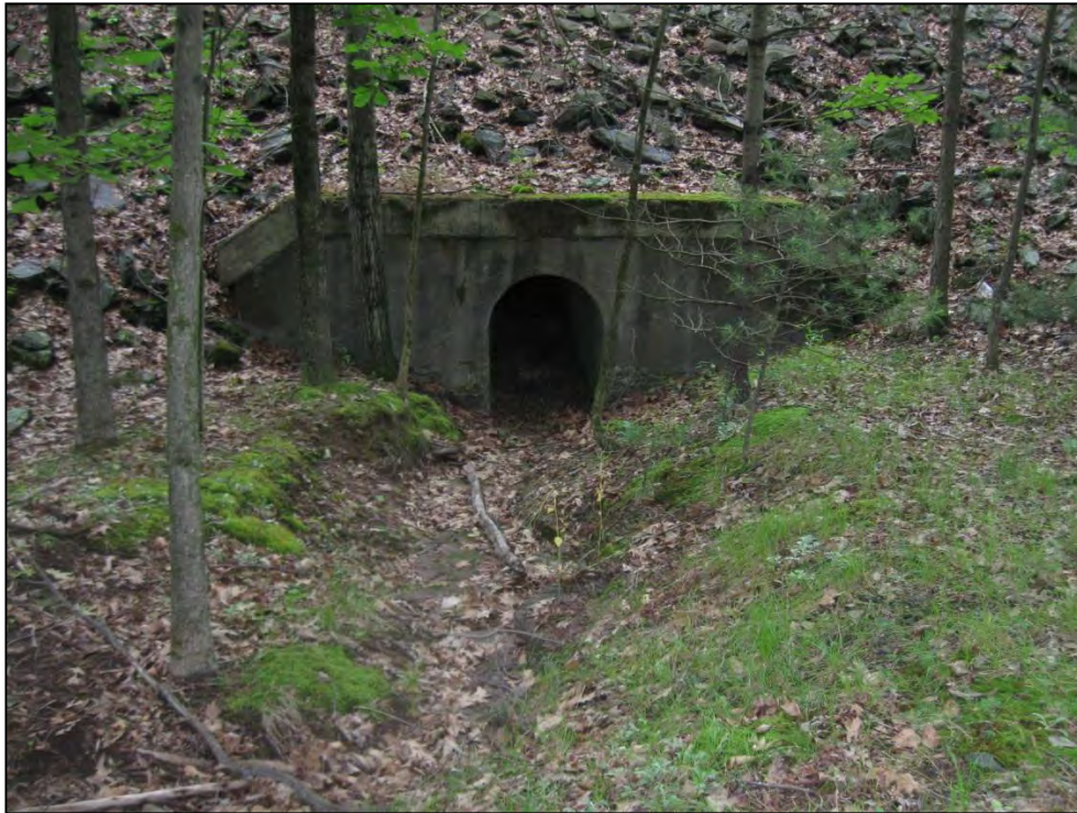
Photo 16. Typical culvert under rail.
