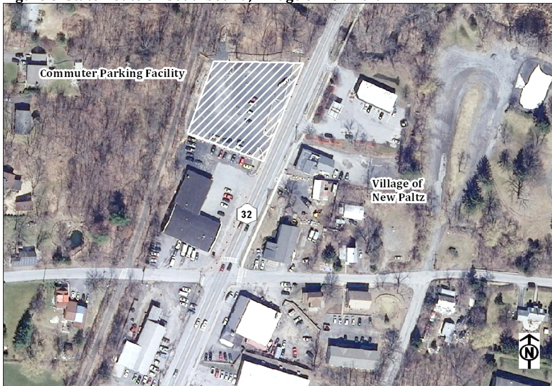
Figure 8: State Route 32 Southbound, Village of New Paltz
