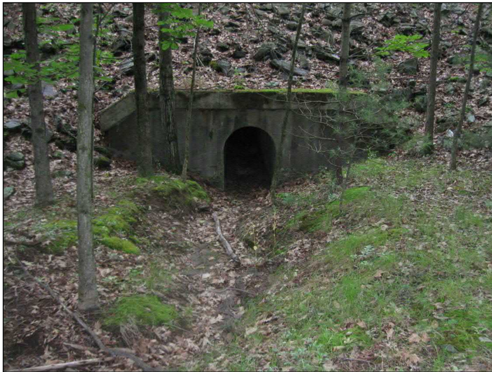
Photo 16. Typical culvert under rail.
