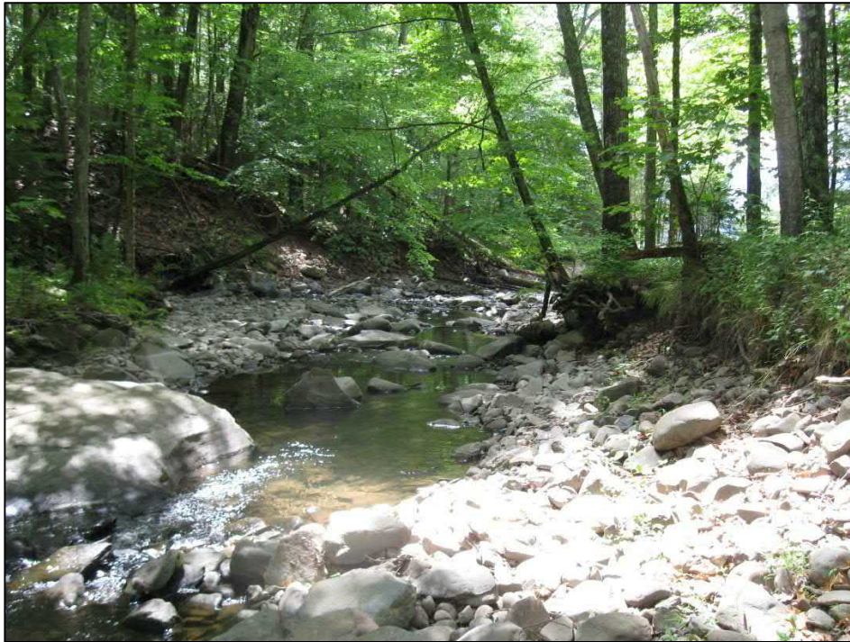
Photo 20. Butternut creek, looking south from failed culvert.
