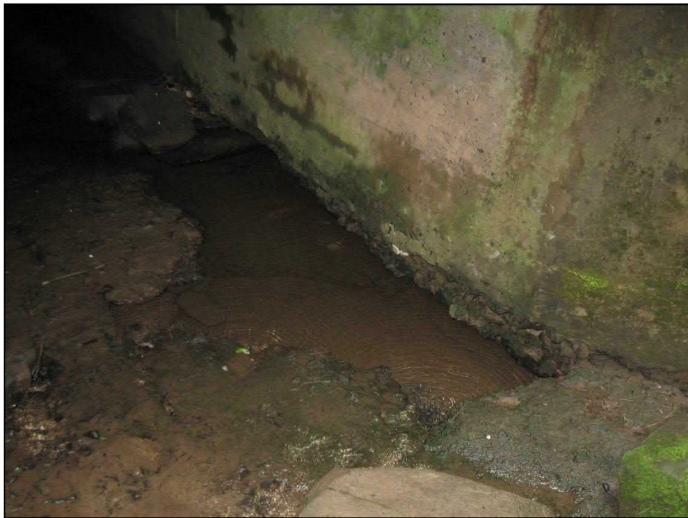
Photo 18. Flow of stream through large culvert.
