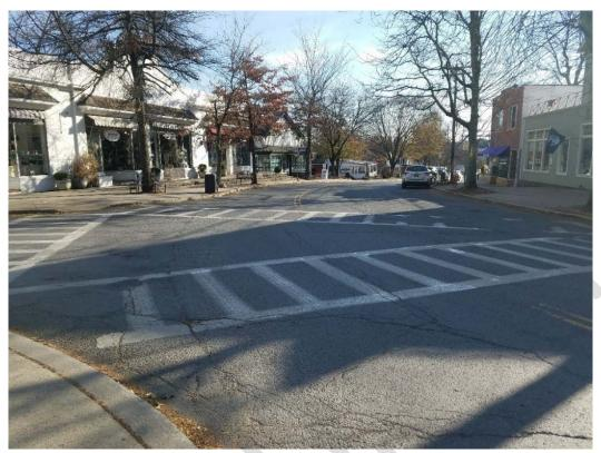
**Photo 1:** View of faded pavement markings and diagonal crosswalks at Rock City Road.
