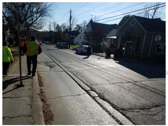
Photo 3: Poor pavement condition in area were trench drain is present.
