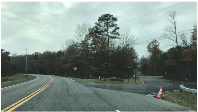
Photo 10: Tight right turn radius at Gate House Road (in vicinity of traffic cone).
