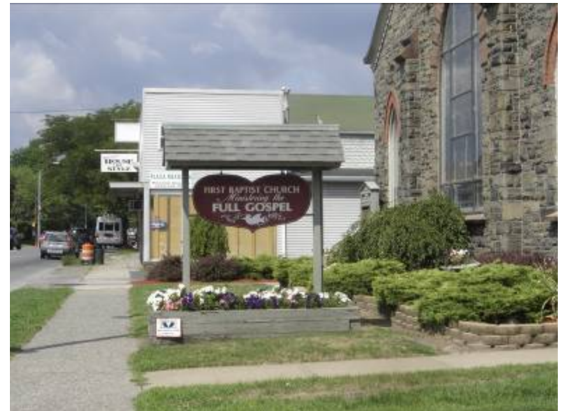
Church driveway too close to intersection
