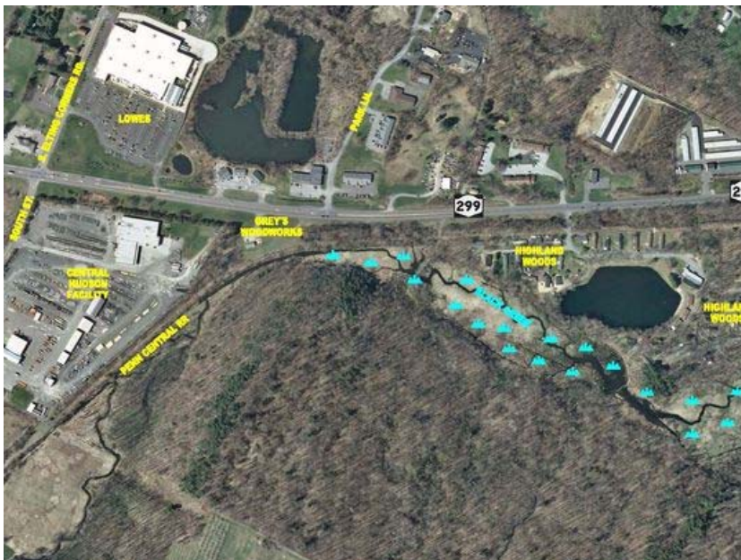
This image provided by HVEA Engineers shows Route 299, alongside which will be a 1.24 mile extension to the Hudson Valley Rail Trail in Highland (Photo: Courtesy of HVEA Engineers)
