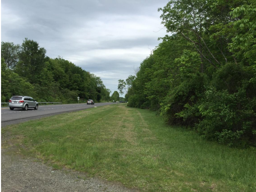
Photo 3 - This picture was taken looking east on the south side of Route 299 at the corner of the hunting club access road.
