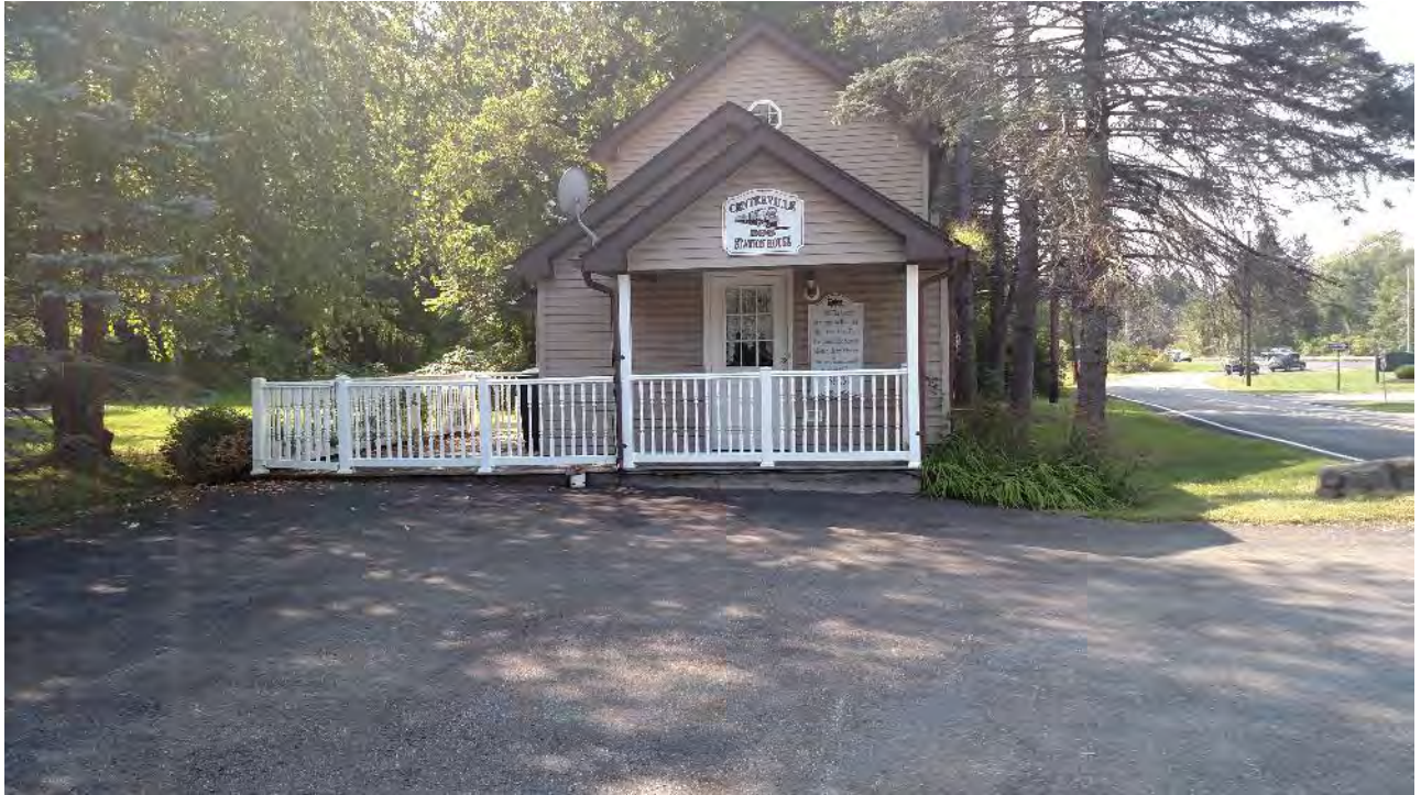
Photo 19: Late 19 th century structure is located adjacent to the eastern terminus of the project corridor. The sign on the building indicates it was built in 1893, and served as Centerville Station. This structure will not be impacted by the proposed project. View to the north. .
