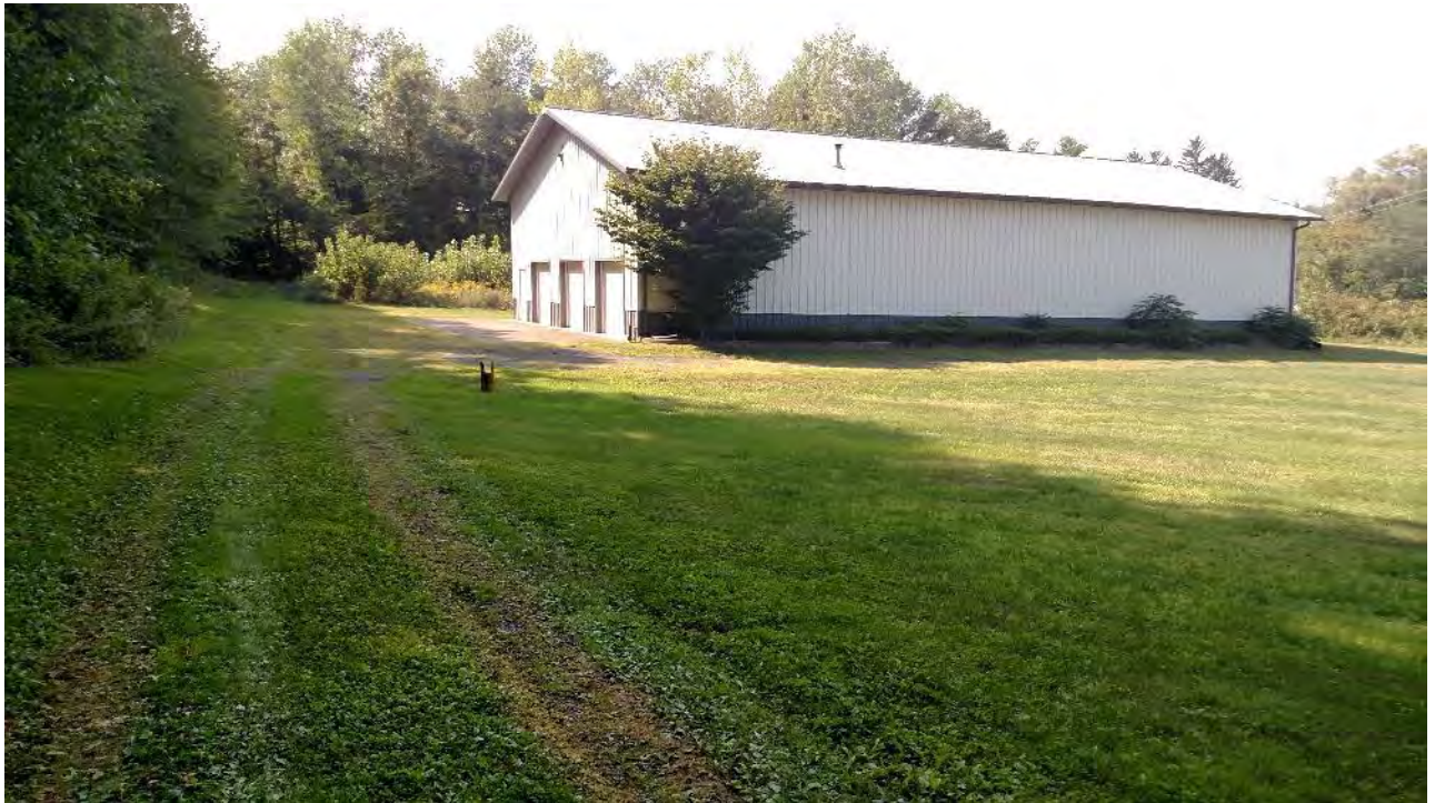
Photo 18: A large concrete and fabricated steel structure is located adjacent to the eastern portion of the project corridor. View to the northwest.
