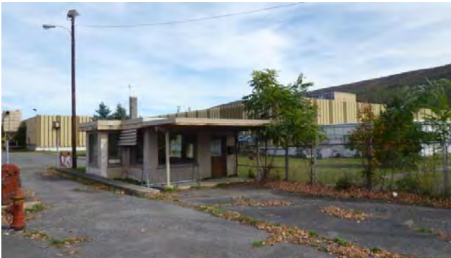
Former Imperial Schrade building
