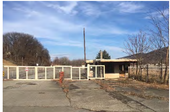
Current entrance to property at Schrade Court, building demolished
