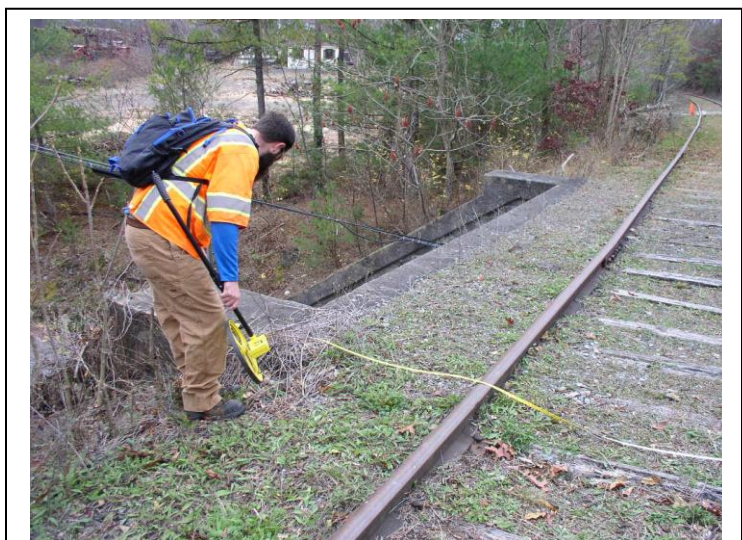
Beesmer Road Bridge
