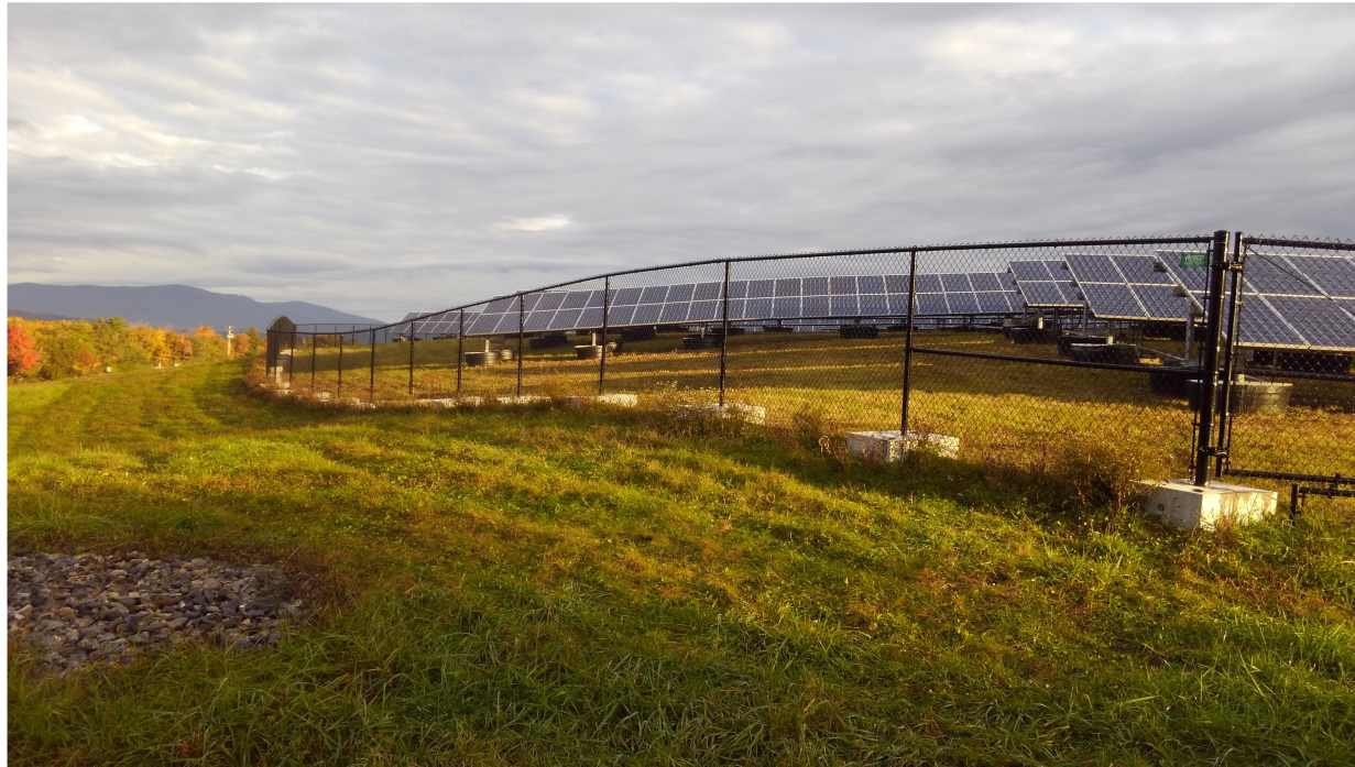
Solar panels at the former Ulster Landfill site
