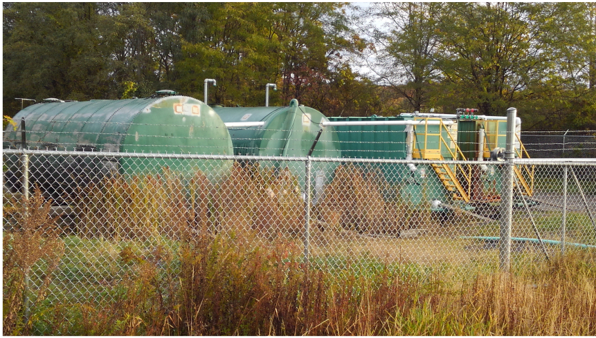
Tanks holding leachate (liquid that drains from landfills)
