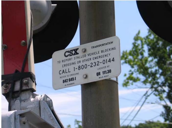
**Figure 3-1. Most grade crossings in the Corridor – and all signalized ones – show the seven-character Association of American Railroads/Federal Railroad Administration crossing ID (lower left). The CSX milepost designation (lower right) is also shown, along with the CSX line designation for the River Line, which is “QR”. This example is at Browns Crossing Road in Catskill.**
