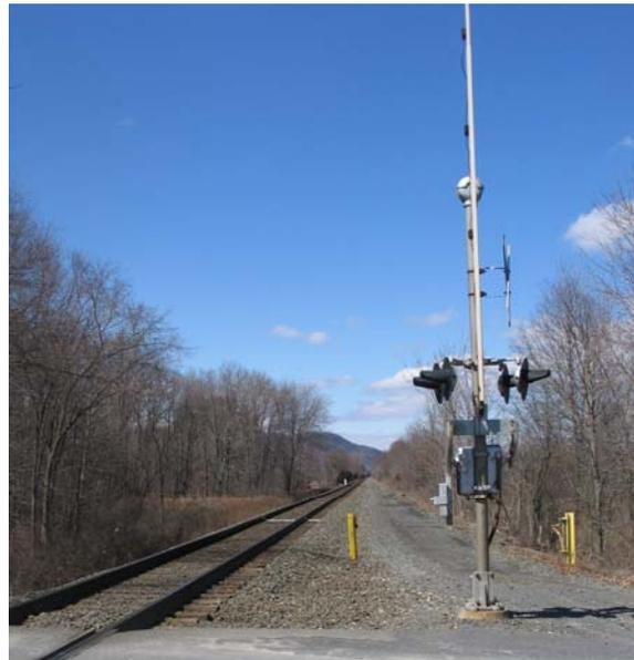
**Figure 3-3. Crossing equipped with gates, flashers and gong at Esopus Avenue. The former two-track alignment of the River Line is evident in this photo.**
