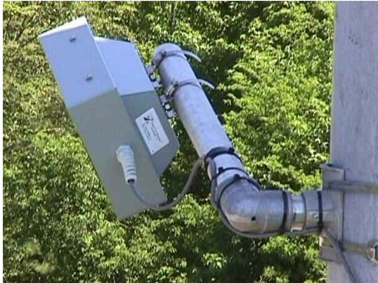
**Figure 6-1: SmarTek Systems – Acoustic Sensor – SAS-1**
