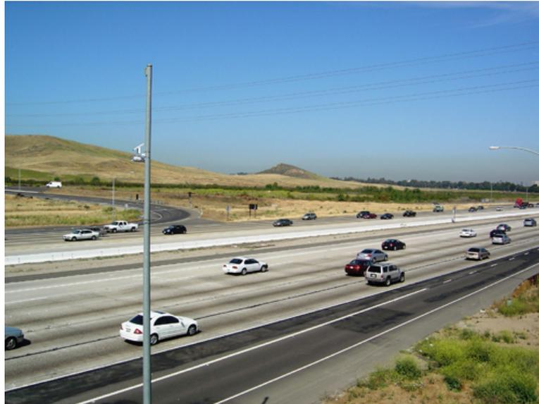
**Figure 6-5: Pole mounting arrangement of SpeedInfo Doppler Radar Speed Sensor DVSS-100**
