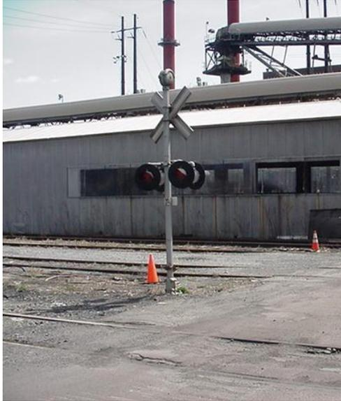
**Figure 3-4. Crossing equipped only with flashers and gong (bell above the crossbucks) at the Danskammer Power Station in Newburgh, Orange County.**
