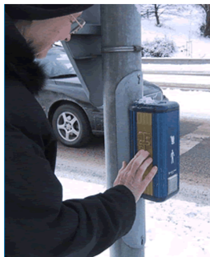
A woman in Sweden uses a tactile map on the side of this APS device to find out what to expect as she crosses the intersection.
