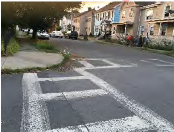
Photograph 1 – Sight distance looking left (D L ) from the west leg of Franklin Street
