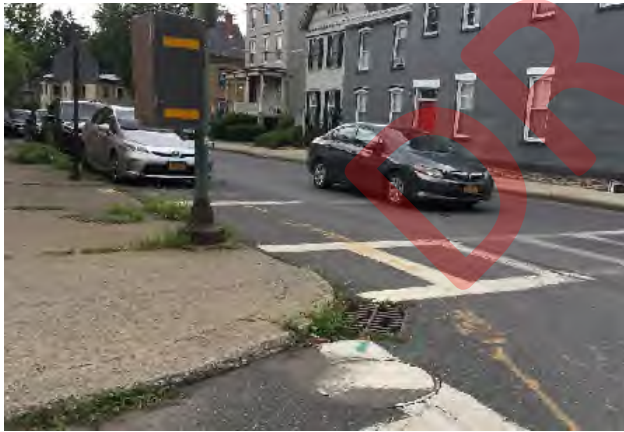
Photograph 1 – Sight distance looking left (D L ) from the south leg of Wall Street
