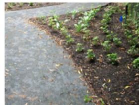
**COMPACTED CRUSHED STONE CONNECTOR**
