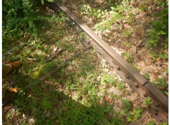
4.8 Defect Tie Condition (§213.109(e) (1))
