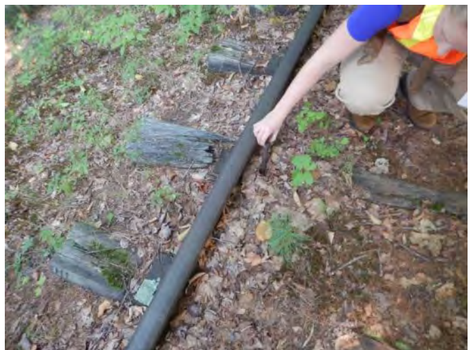
4.24 Defective Tie, Tie Unable To Hold Spike (§213.109(c) (2))
