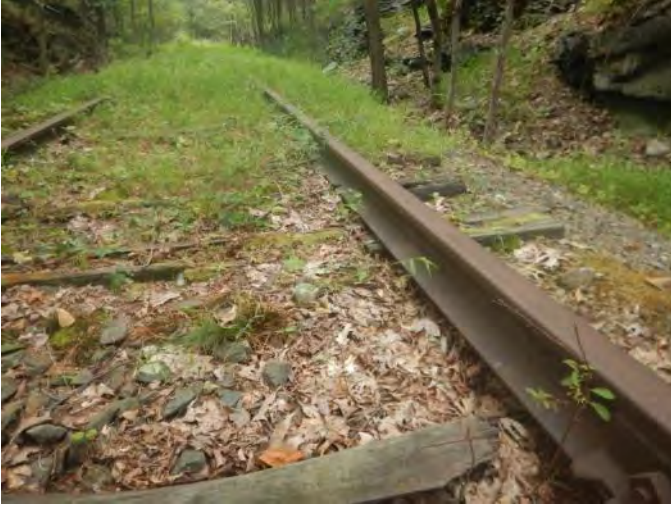
4.7 No Effective Support Ties Within The Prescribed Distance From A Joint (§213.109(e) (1))
