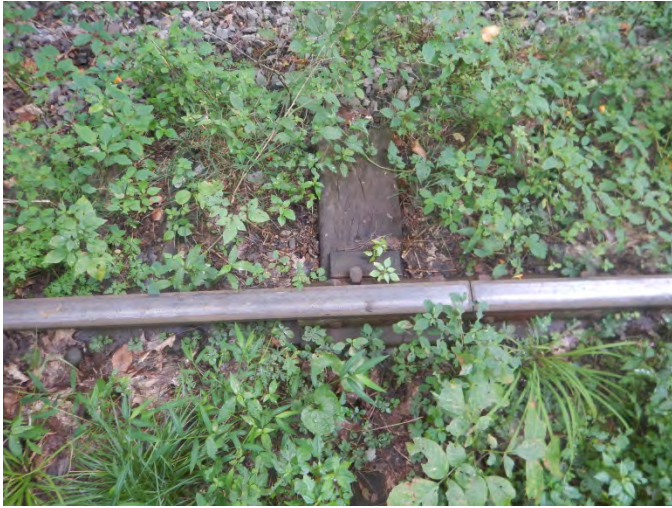
8.1 Tie Condition Generally Meets Class 1
