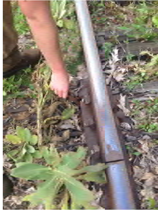
9.2 Defective Tie, Tie Unable To Hold Spike (§213.109(c) (2))
