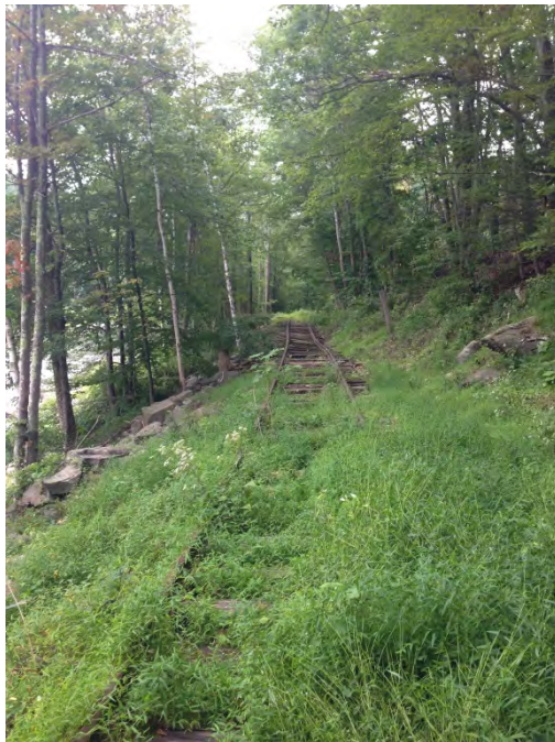
7.3 Washout, Insufficient Ballast (§213.103(a))
