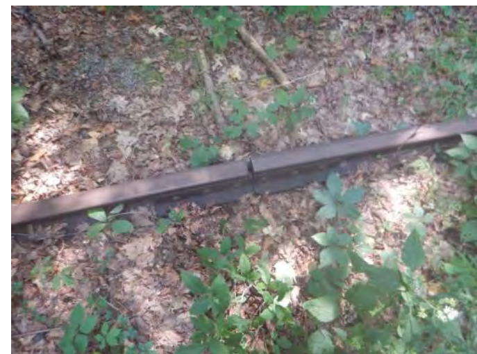
4.12 Center Cracked Joint Bar (§213.121(c))
