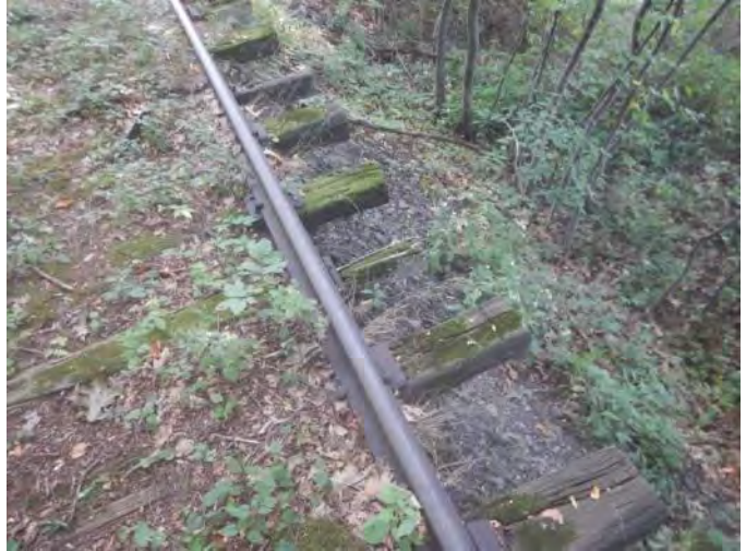
4.14 Poor Tie Condition and Insufficient Ballast (§213.109(e) (1) and §213.103(a))
