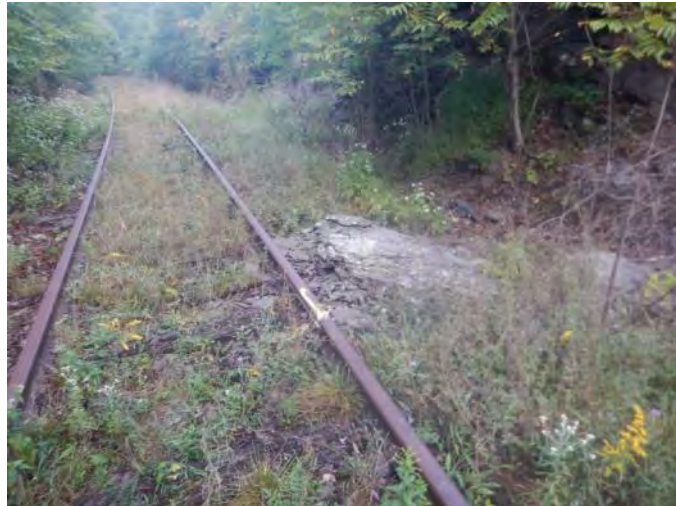
4.4 Rockslide Next To Joint Tie Defect (§213.109(e) (1))
