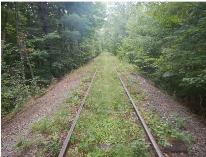
8.3 Tie Condition Generally Meets Class 1, Vegetation Defects Observed (§213.37)
