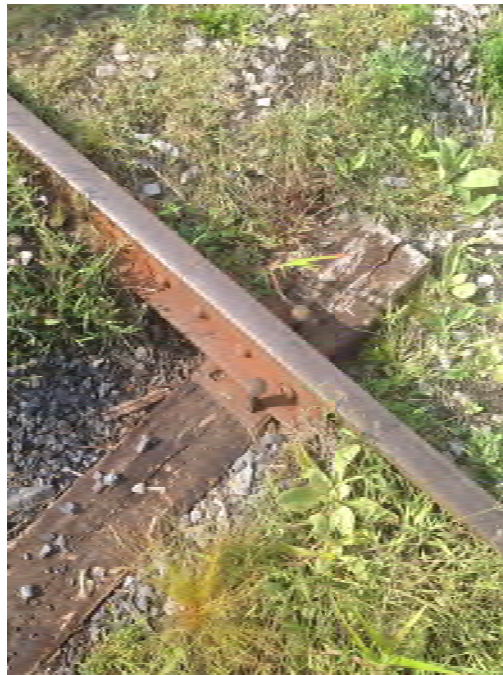
1.2 Tie Condition Observed
