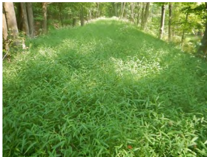
4.11 No Vegetation Management (§213.37), Difficult To Inspect
