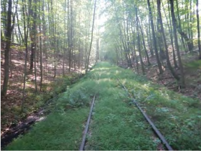
4.13 Poor Drainage And No Vegetation Management (§213.33 And §213.37)
