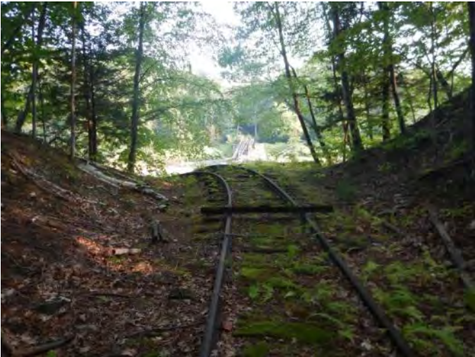
5.2 Poor Tie Condition On Espous Creek Trestle Approach (§213.109(e) (1))
