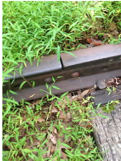
7.4 Center Cracked Joint Bar (§213.121(c))
