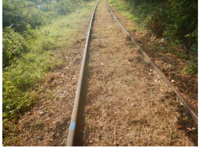
2.2 Tie Condition Generally Meets Class 1
