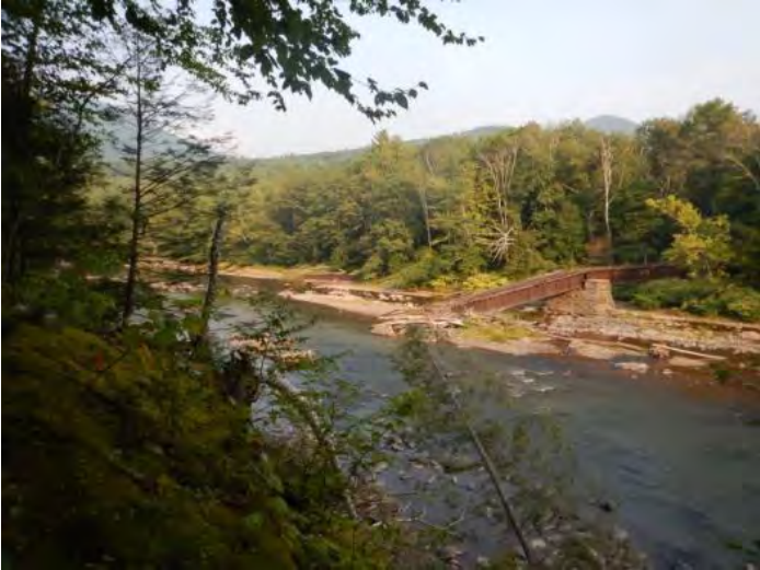
5.1 Failed Esopus Creek Trestle
