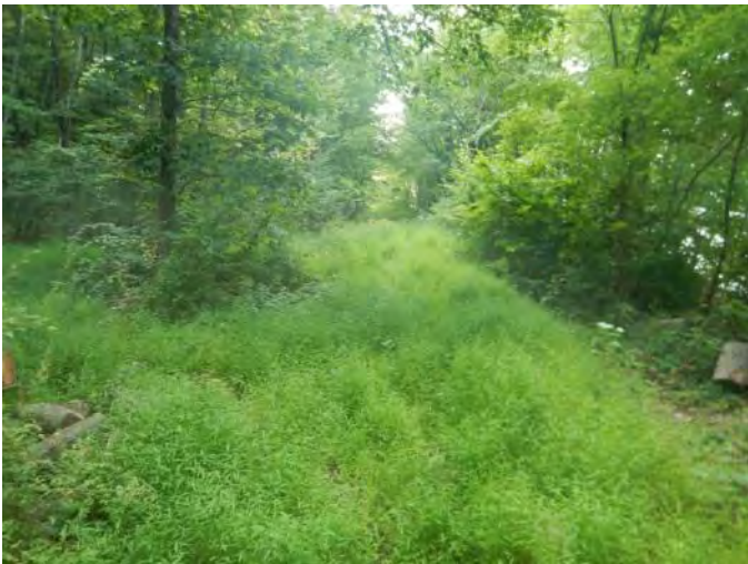
4.21 No Vegetation Management (§213.37), Difficult To Inspect
