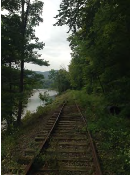
7.1 Washout, Insufficient Ballast (§213.103(a))
