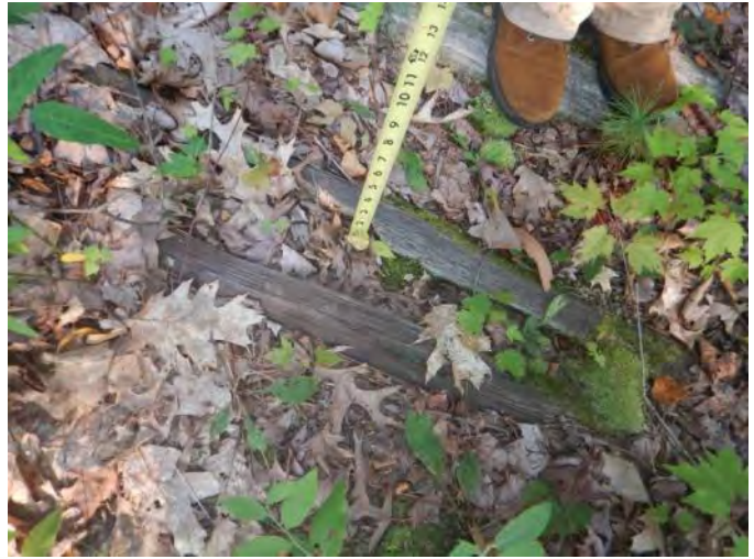
4.20 Detailed View of Deteriorated (§213.109(c) (3))
