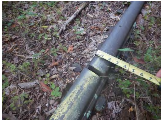
4.18 Rail End Mismatch (§213.115)
