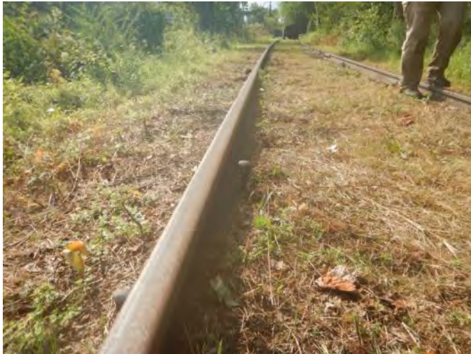
2.3 No effective supports ties within the prescribed distance from a joint (§213.109(e) (1))
