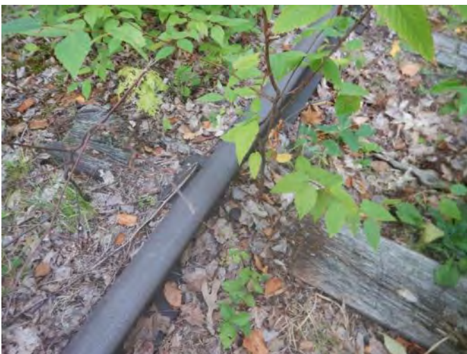
4.23 Defective Tie, Vegetation Growing Through Tie (§213.109(c) (2))
