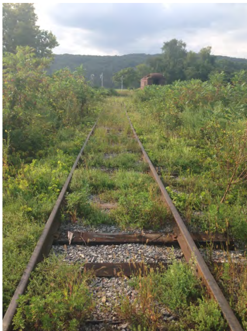
1.4 Tie Condition Generally Meets Class 1
