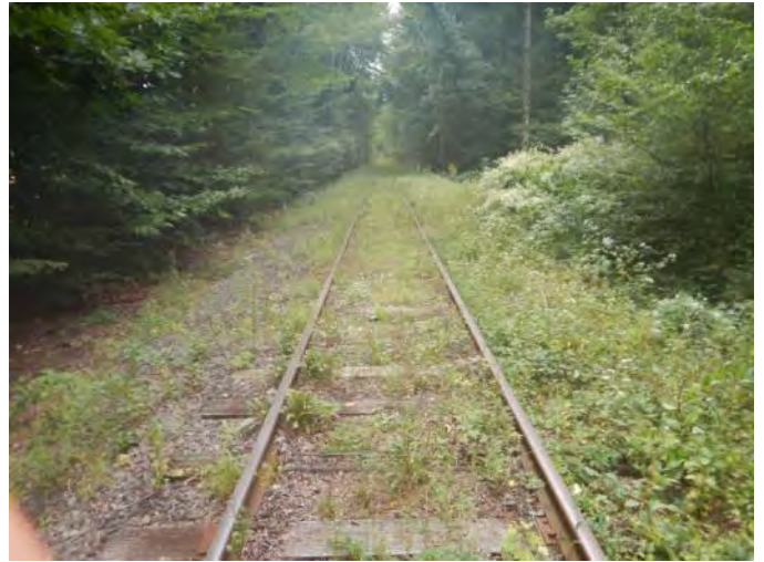
8.2 Tie Condition Generally Meets Class 1, Vegetation Defects Observed (§213.37)
