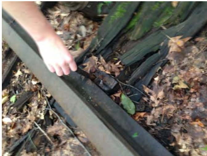
6.3 Defective Tie, Tie Unable To Hold Spike (§213.109(c) (2))
