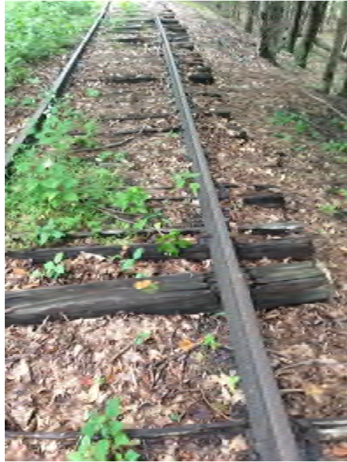
6.2 No Effective Support Ties Within The Prescribed Distance From A Joint (§213.109(e) (1))
