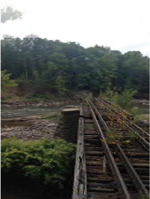
5.2 Poor Timber Condition On Espous Creek Trestle Approach (§213.109(e) (1))
