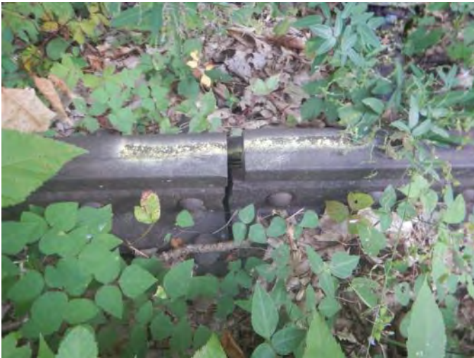
4.19 Previously Marked Center Cracked Joint Bar – Defect Not Addressed (§213.121(c))
