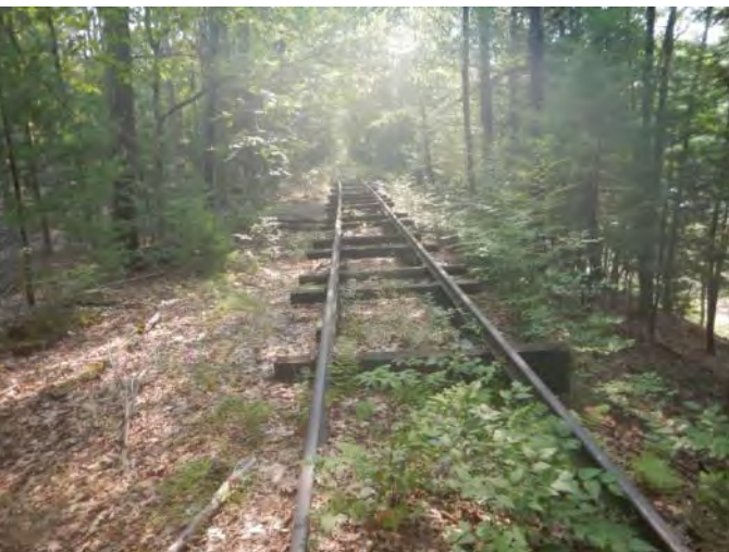
4.17 Washout, Insufficient Ballast (§213.103(a))
