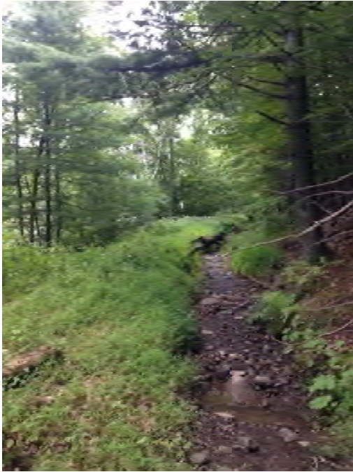
6.1 Poor Drainage And No Vegetation Management (§213.33 And §213.37)
