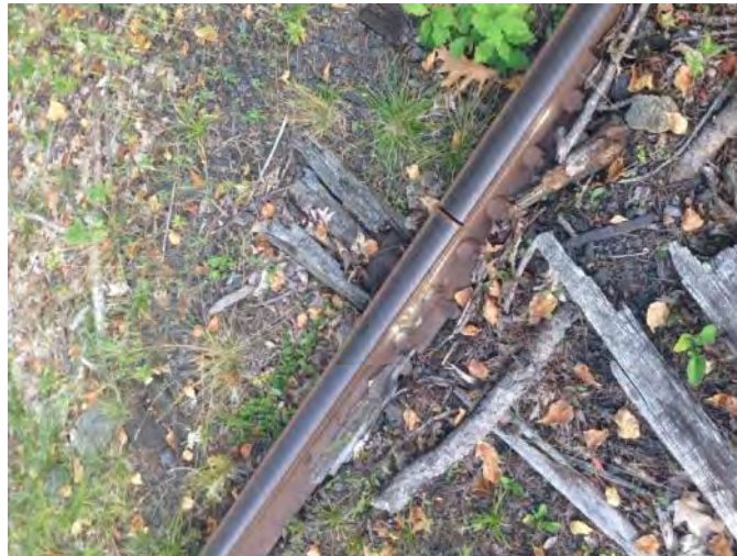
9.3 No Effective Support Ties Within The Prescribed Distance From A Joint (§213.109(e) (1))
