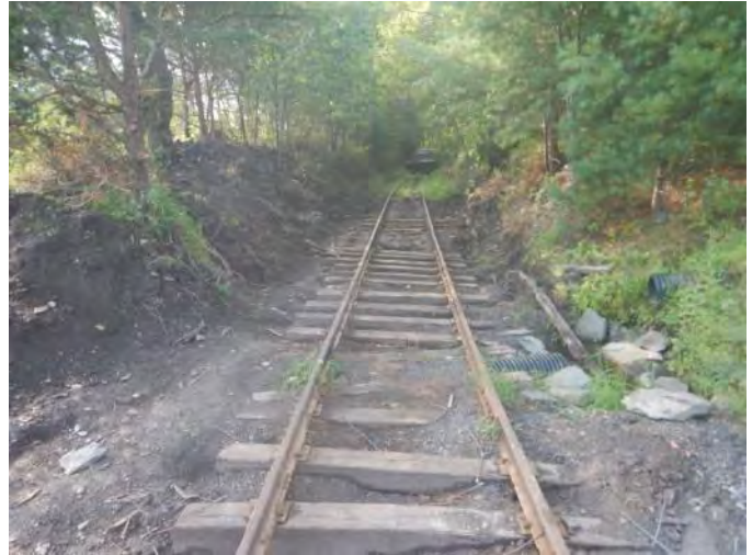
2.4 Tie Condition Generally Meets Class 1. Insufficient ballast (§213.103(a))
