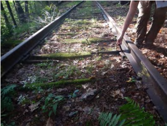
4.3 Defective Tie, Tie Unable To Hold Spike (§213.109(c) (2))
