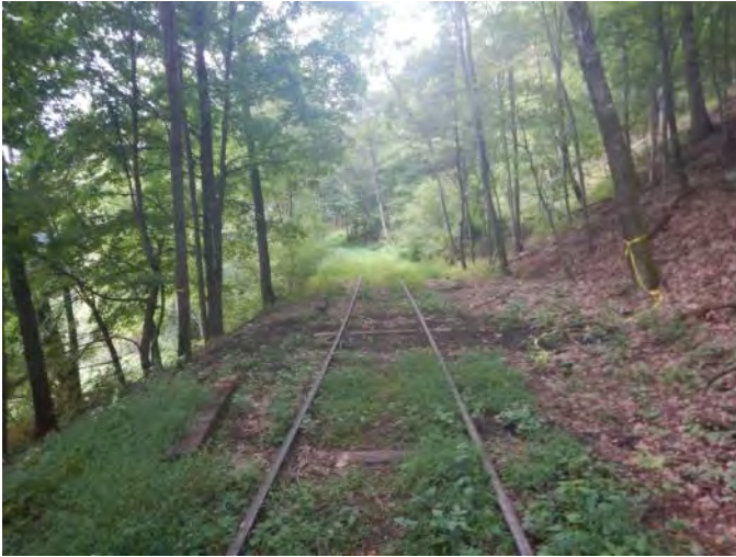
3.1 Recently Changed Ties To Meet Class 1. No Vegetation Management ($213.37)
