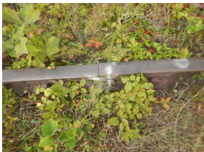
4.6 Previously Marked Center Cracked Joint Bar – Defect Not Addressed (§213.121(c))
