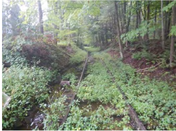
4.2 Poor Drainage And Defective Tie Condition (§213.33 and §213.109(e) (1))
