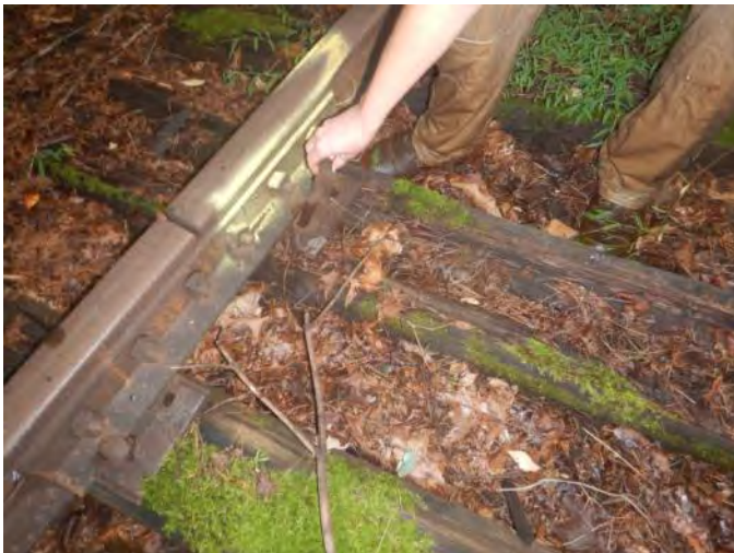
4.5 Previously Marked Joint Tie Defect, Tie Unable To Hold Spike – Defect Not Addressed (§213.109(c) (2))
