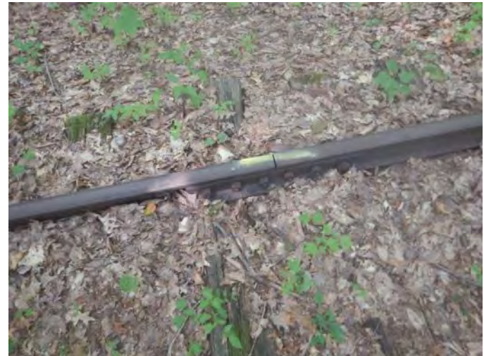
4.10 Previously Marked Joint Tie Defect, Tie Unable To Hold Spike – Defect Not Addressed (§213.109(c) (2))
