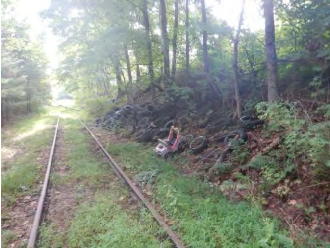
4.1 Previously Observed Tire Pile. Right Of Way Was Not Free Of Brush, Litter And Debris.
