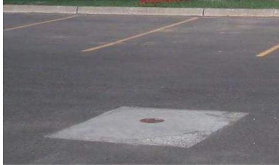
Flush mount in pavement (square conc. patch is common)
