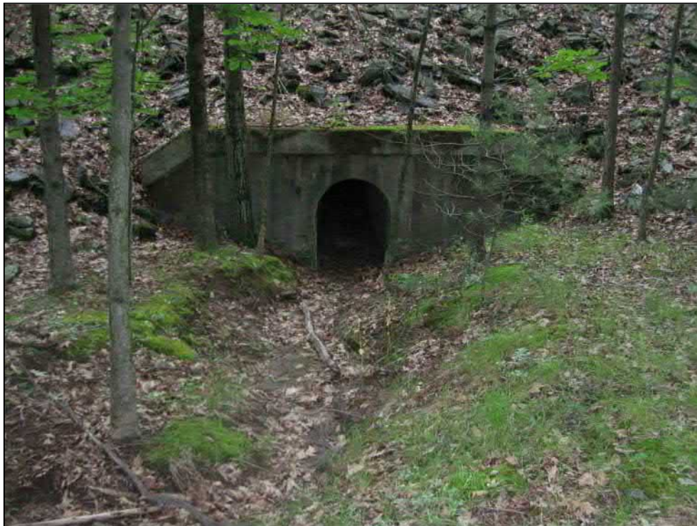
Photo 16. Typical culvert under rail.
