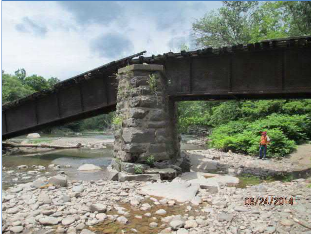
View Looking at Existing Pier 1 (Span 1 on Pier, Span 2 Resting on Ground): Boiceville Trestle
