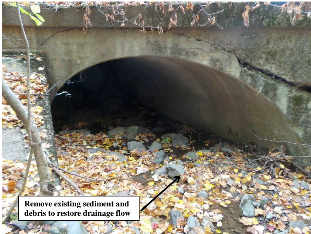
Upstream Invert conditions: Culvert #36
