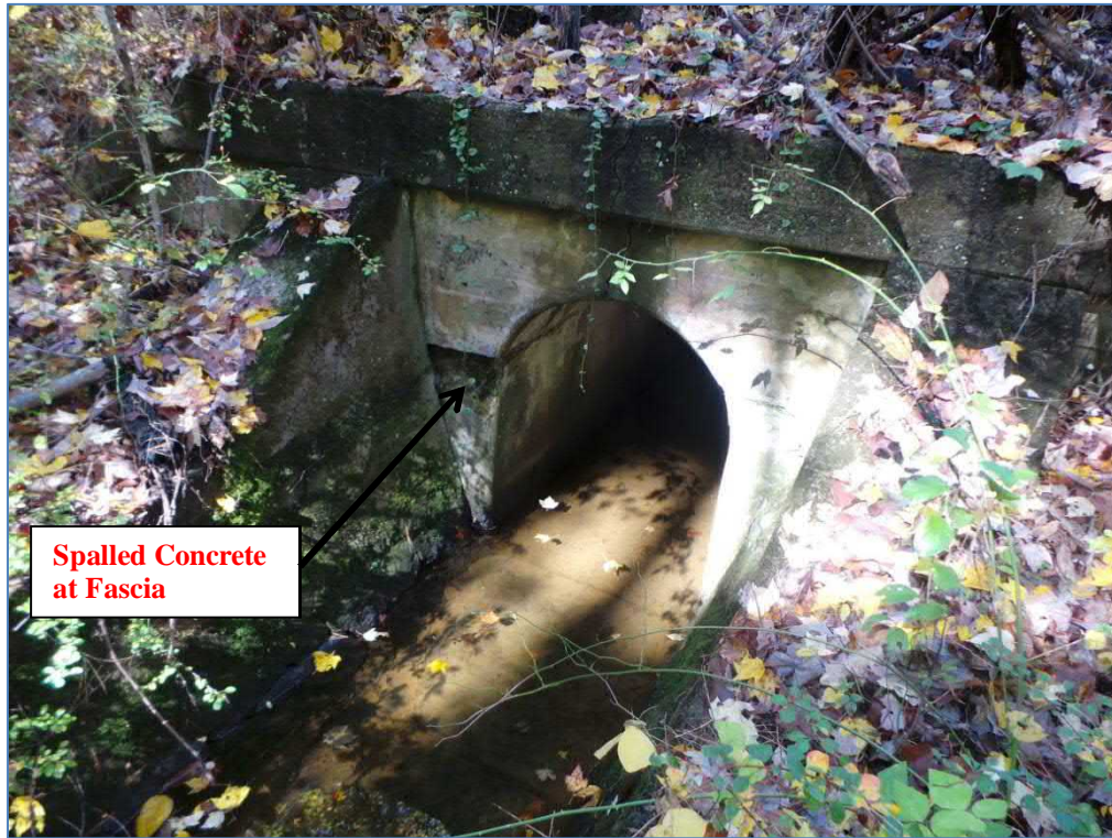
Downstream Culvert Fascia: Culvert #23
