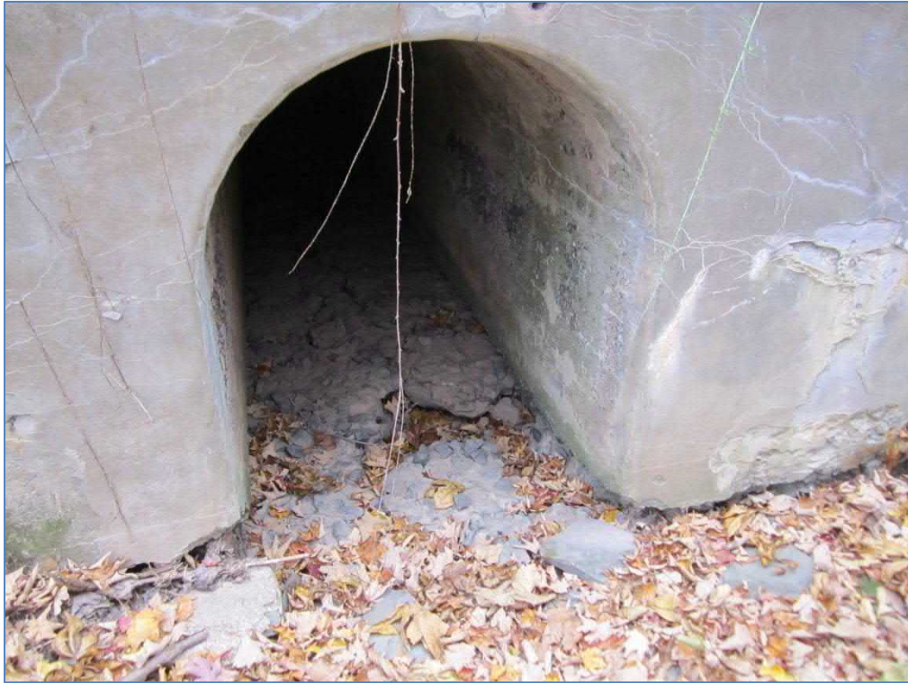
View of Upstream Scour at Concrete Bottom Slab: Culvert #4
