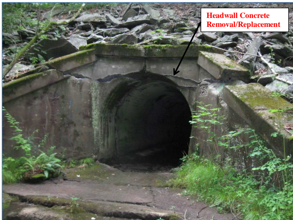
Downstream Culvert Elevation: Culvert #7
