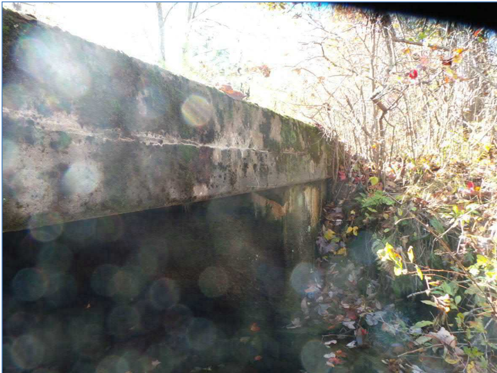
Cracks in Concrete Headwall: Culvert #24
