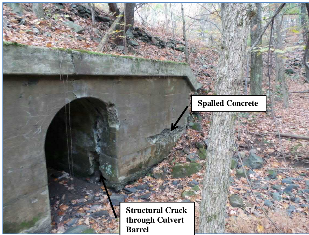
General View of Existing Deterioration: Culvert #3
