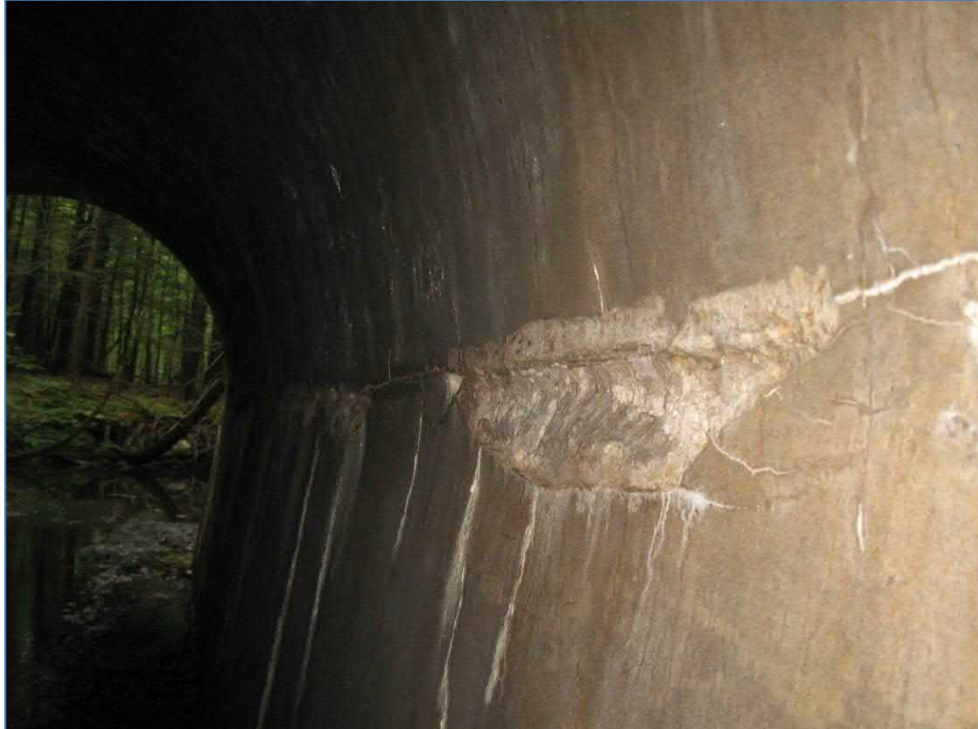
Spalled Concrete Inside Culvert Barrel: Culvert #12
