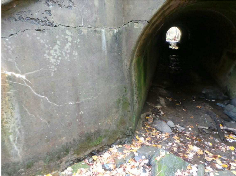
Scour/Erosion at Downstream Wingwall Apron: Culvert #7
