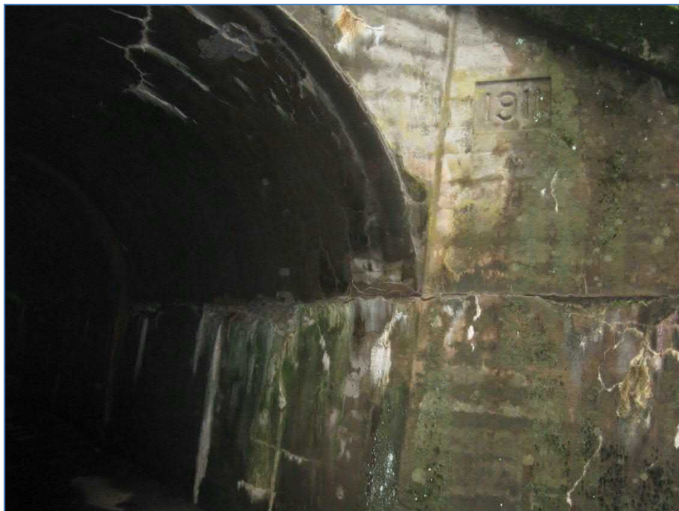
Cracked Concrete at Wingwalls: Culvert #12
