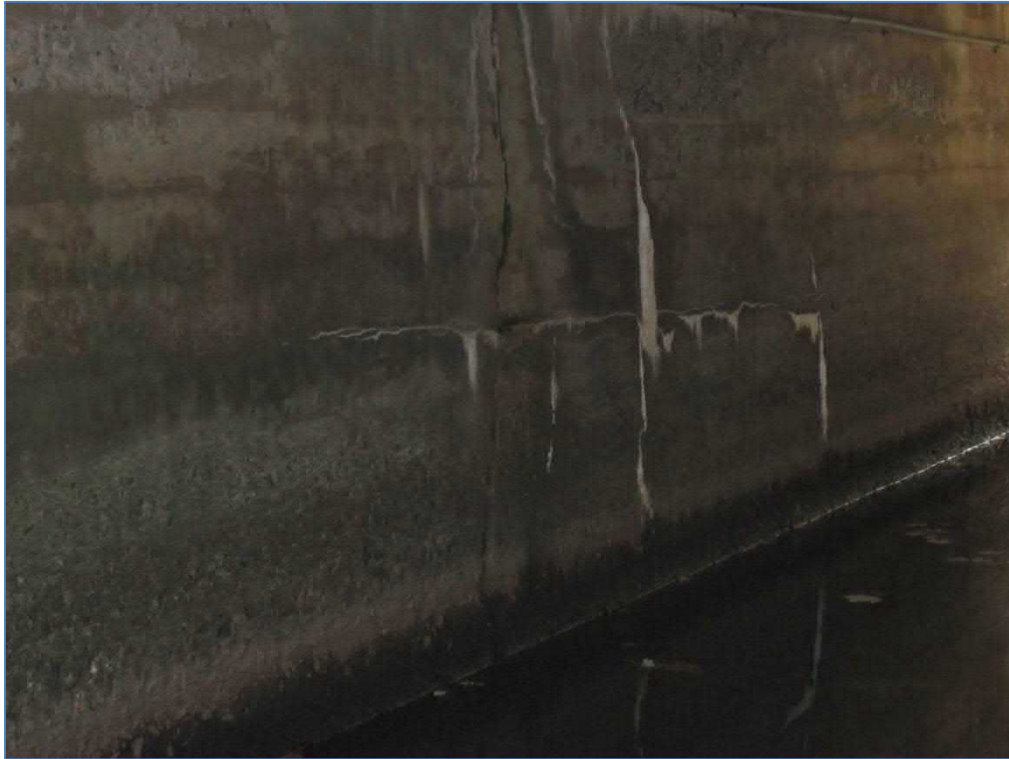
Cracks in Vertical Wall of Culvert: Culvert #22
