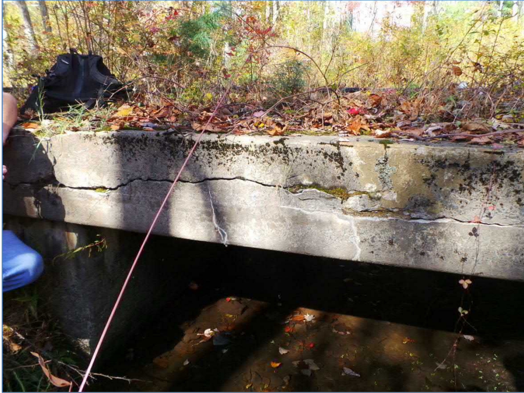
Cracks in Concrete Headwall: Culvert #24
