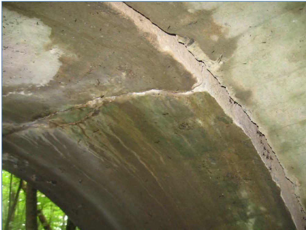
Crack in Culvert Barrel: Culvert #5
