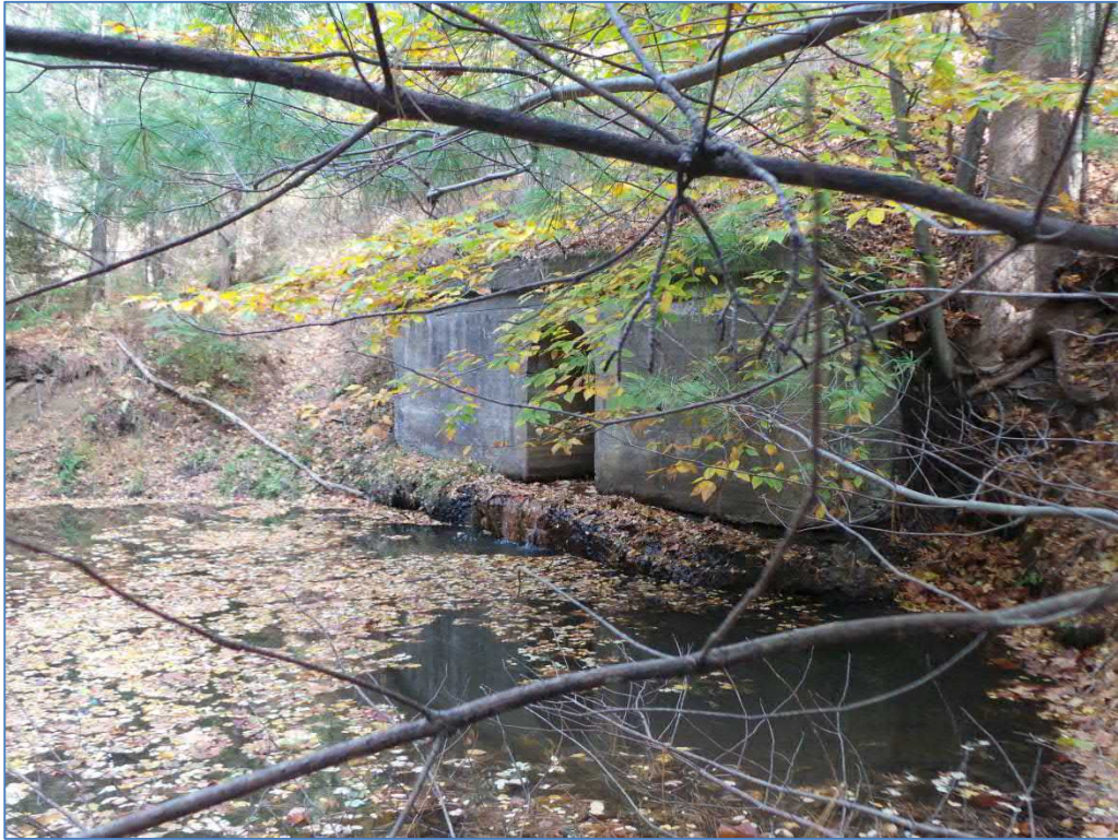
Downstream Culvert Fascia, Showing Drop Off to Stream Bed: Culvert #29
