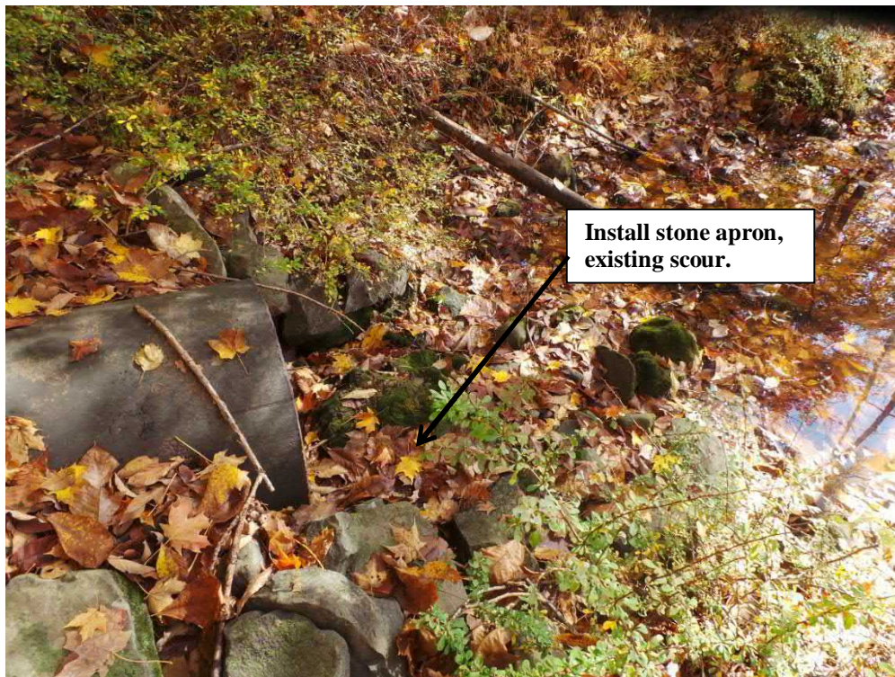
Downstream Culvert Elevation: Culvert #21
