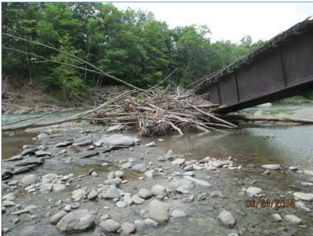
View Looking at End of Span 2 Resting on Creek Bed: Boiceville Trestle
