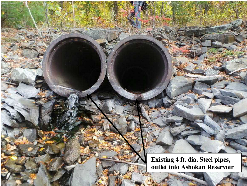
Downstream Elevation: Culvert #35
