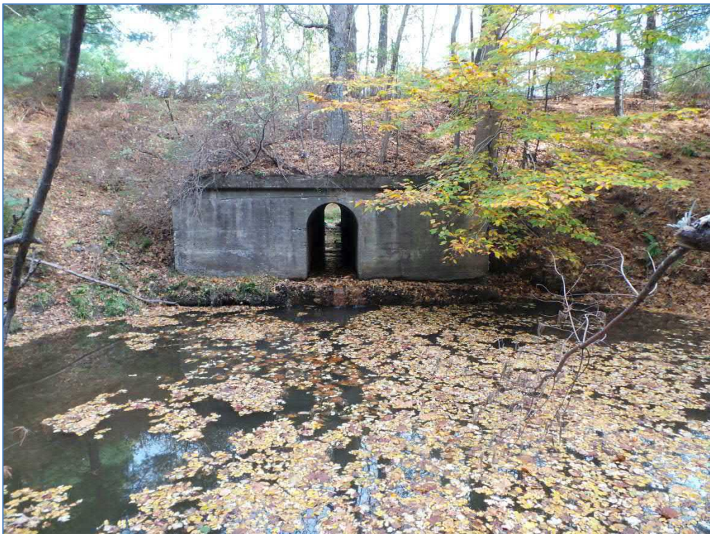
Downstream Culvert Fascia, Showing Drop Off to Stream Bed: Culvert #29
