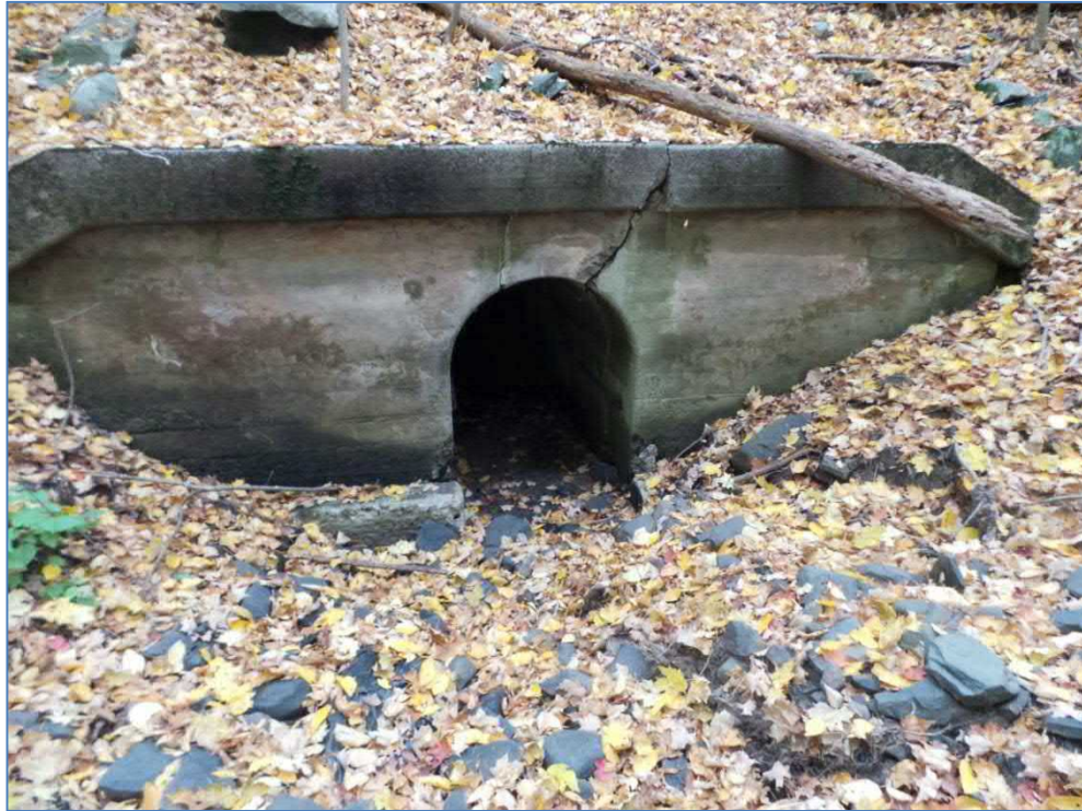
Upstream Culvert Elevation, Showing Existing Cracks: Culvert #19
