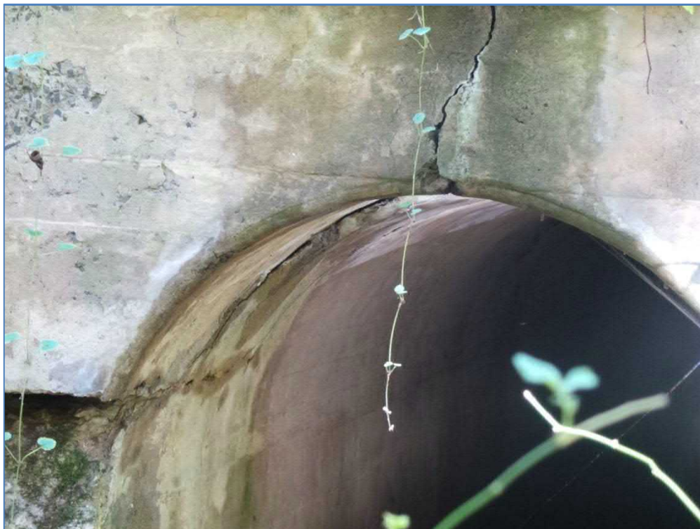
Downstream Culvert Fascia, Showing Cracks in Headwall: Culvert #23
