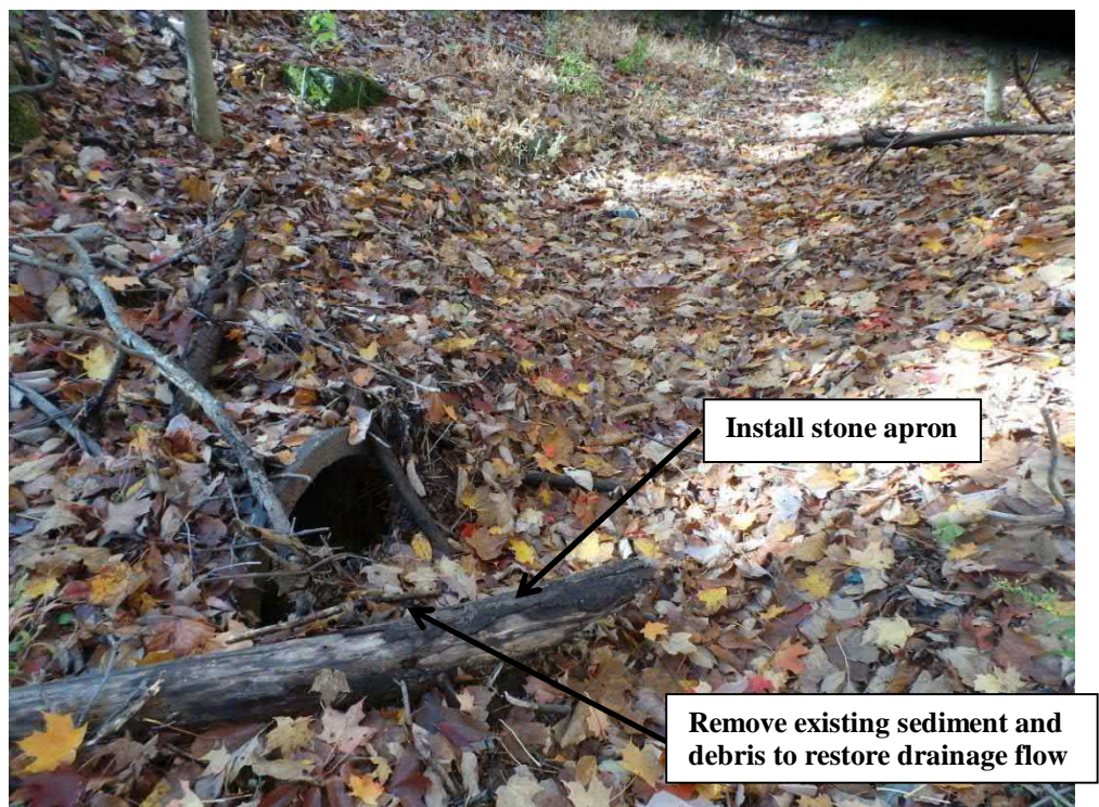
Upstream Culvert Invert conditions: Culvert #21
