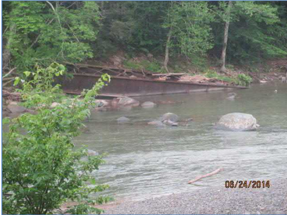
View Looking Towards Girders Resting Along South Stream Bank: Boiceville Trestle
