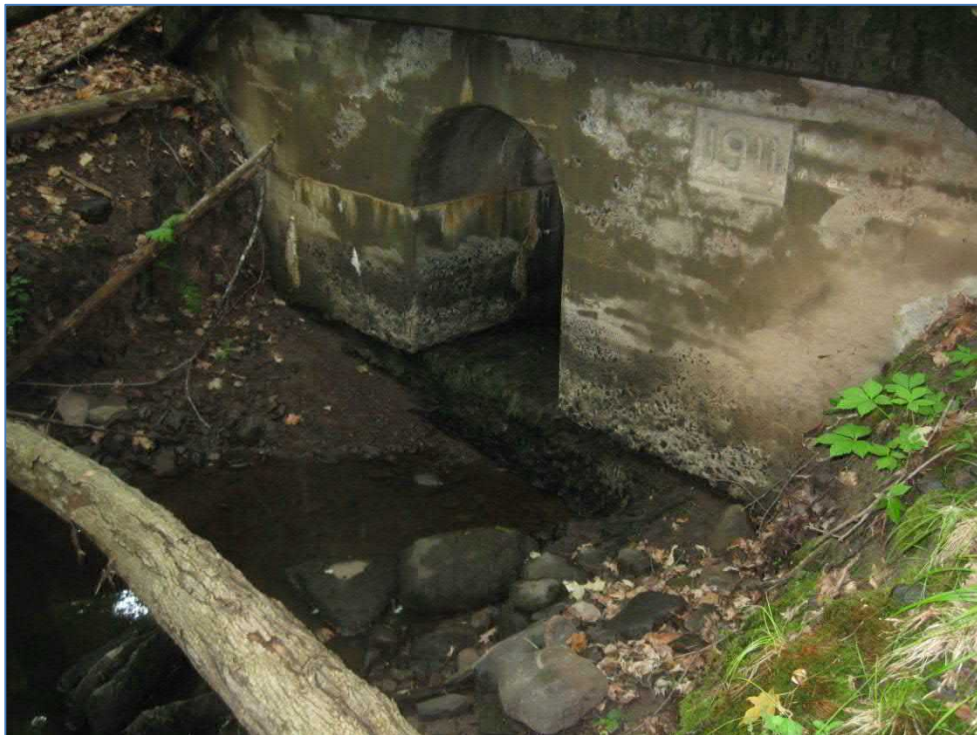
Upstream Culvert Elevation, Showing Existing Cracks: Culvert #19
