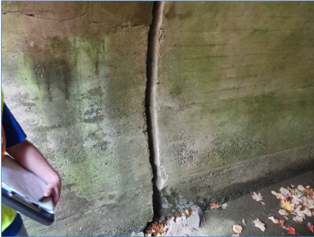
Crack in Culvert Barrel: Culvert #5
