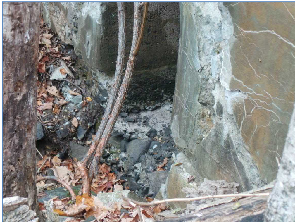
View of Scour at Downstream Culvert Fascia: Culvert #4
