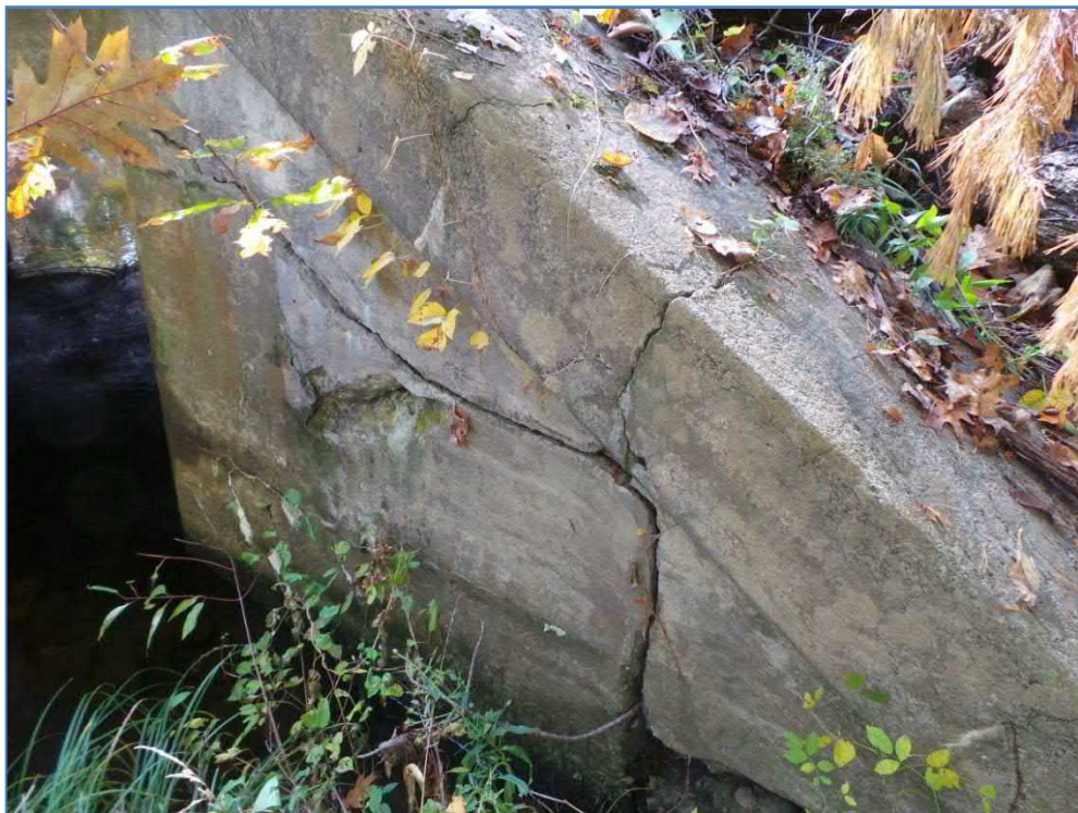
Cracks in Wingwall: Culvert #22
