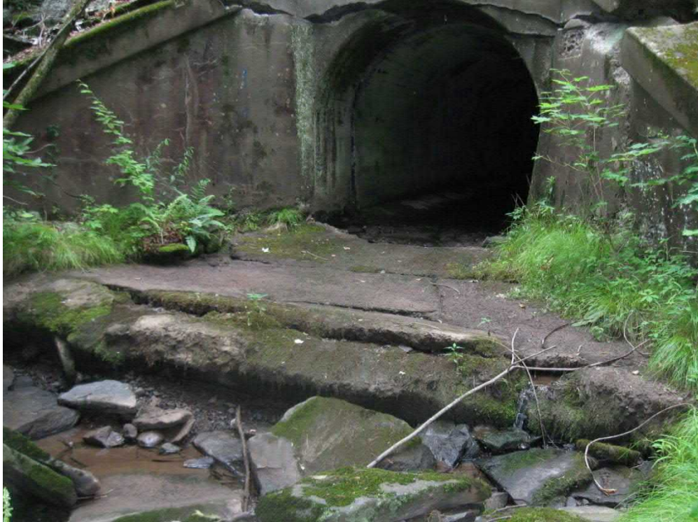
Scour/Erosion at Downstream Wingwall Apron: Culvert #7
