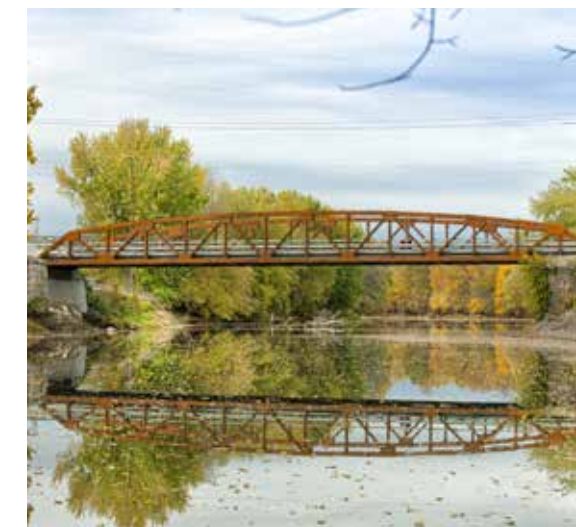
Wynkoop Rd bridge in Hurley.
