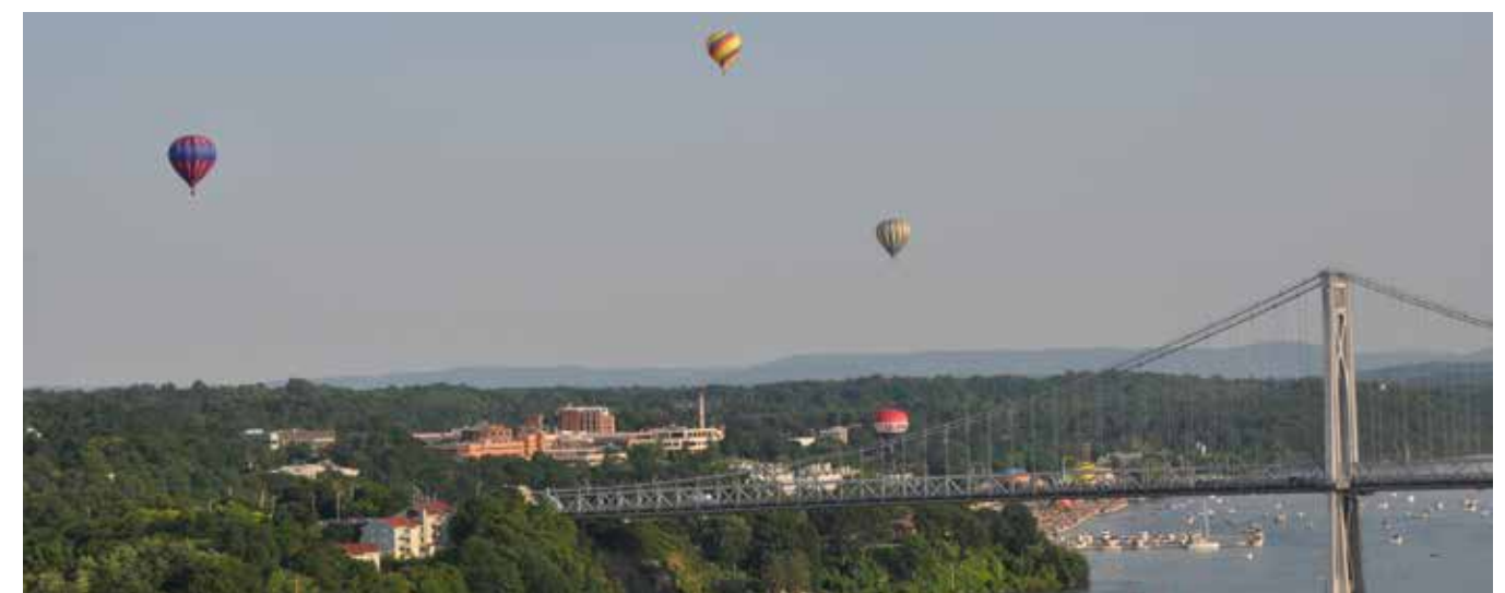
The Mid Hudson Valley Bridge.
