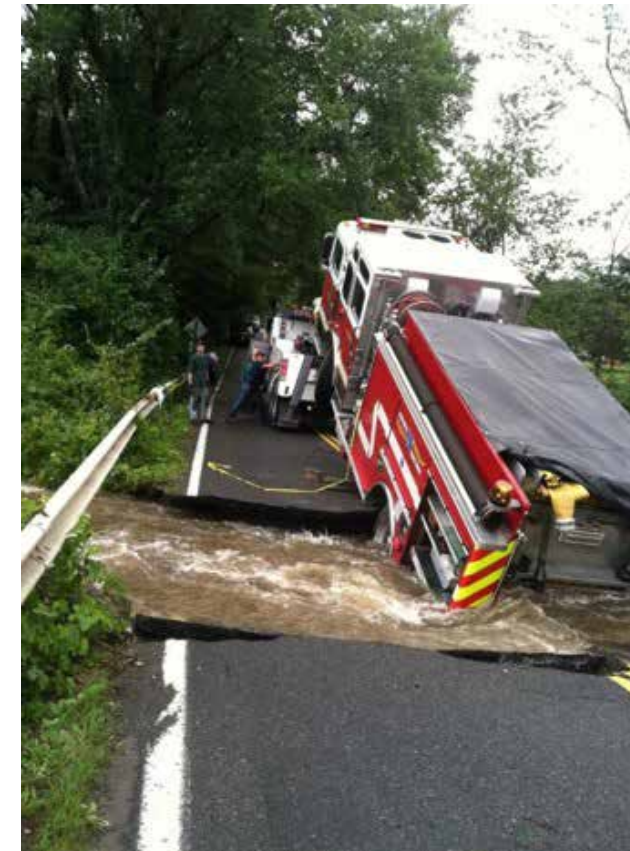
Firetruck being rescued by tow truck from culvert that has collapsed due to severe flooding.
