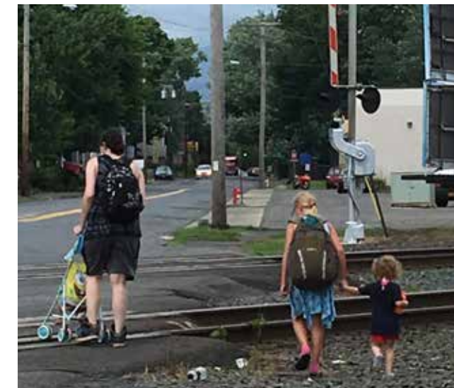
A mother with three children traverses the uneven gap between sidewalk segments at the CSX track on Foxhall Ave. in Kingston. The City of Kingston has secured funding to provide new sidewalks in this location and is working with NYSDOT to secure HSIP Rail funds to improve the crossing. Source: UCTC July 2018.
