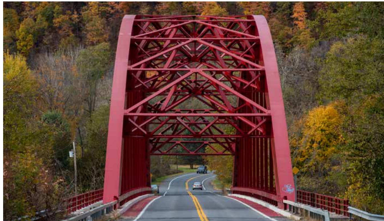
The Eddyville Bridge on Route 213 in Eddyville, NY.
