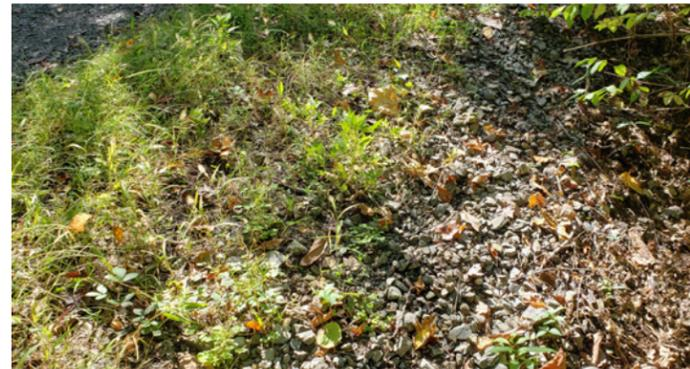
There is exposed ballast stone along the edges of the WVRT. It is likely the ballast stone extends under the existing trail surface.
