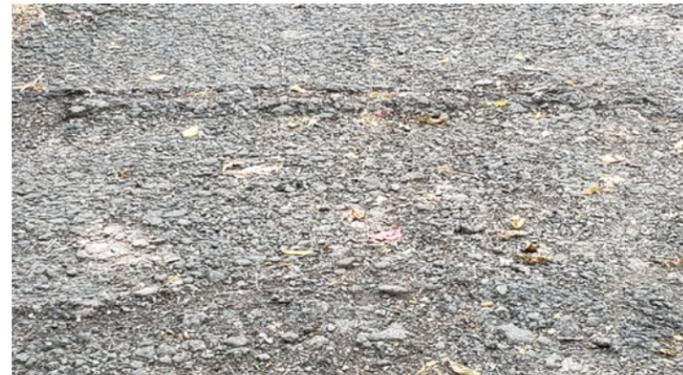
Broken and deteriorated asphalt are compounded by areas of trail surface pushed up the tree roots that occur unexpectedly along the trail.
