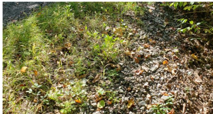
There is exposed ballast stone along the edges of the WVRT. It is likely the ballast stone extends under the existing trail surface.
