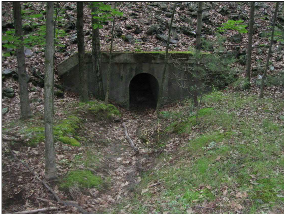
Photo 16. Typical culvert under rail.
