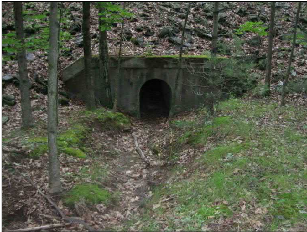
Photo 16. Typical culvert under rail.
