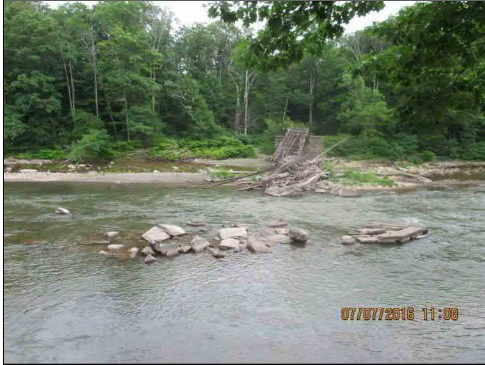
Photo 9. View looking west at proposed Espopus crossing. "Boiceville Trestle" destroyed by Tropical Storms Irene and Lee.
