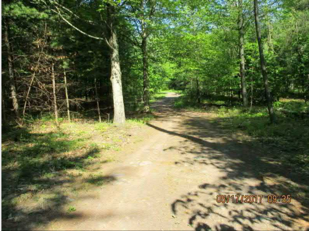
Photo 17. Existing access road, to receive a layer of stone dust.
