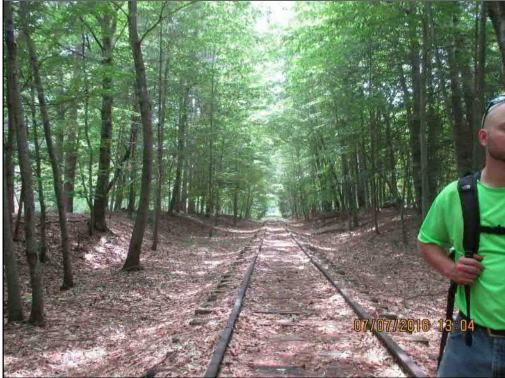
Photo 15. Corridor on western side of Esopus, looking east.
