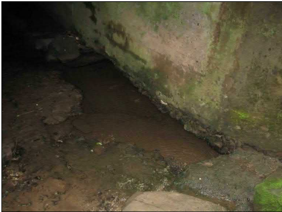
Photo 18. Flow of stream through large culvert.
