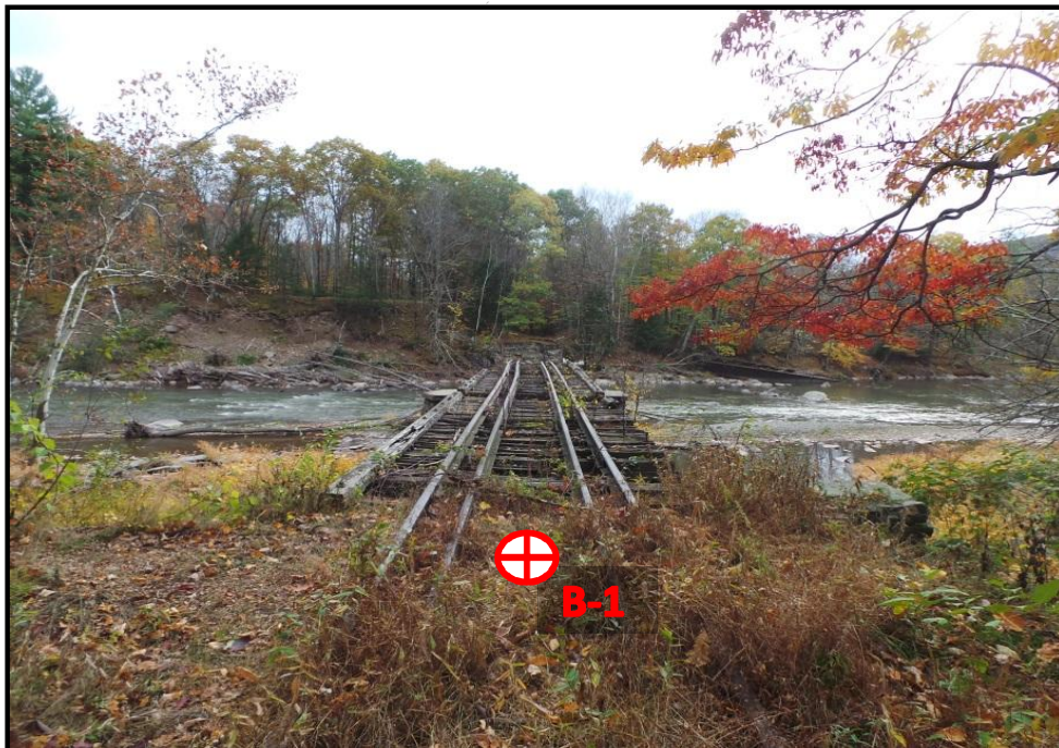
Boring 1: Boiceville Railroad Trestle West Approach
