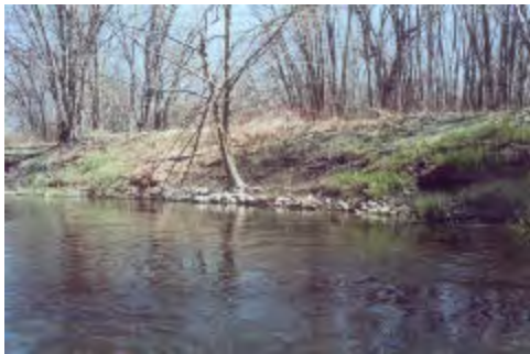
Small rock at the toe of the bank has proven effective on this reach of the Wallkill
