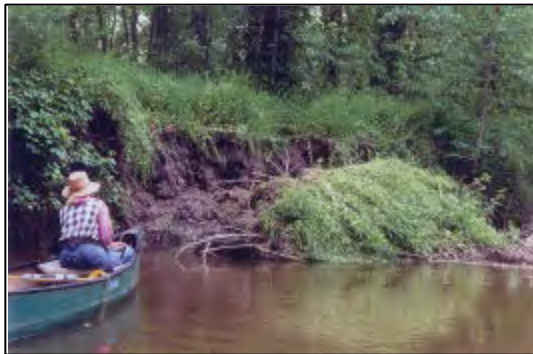
Undercutting of the toe eventually results in huge sections of River bank collapsing into the channel.
