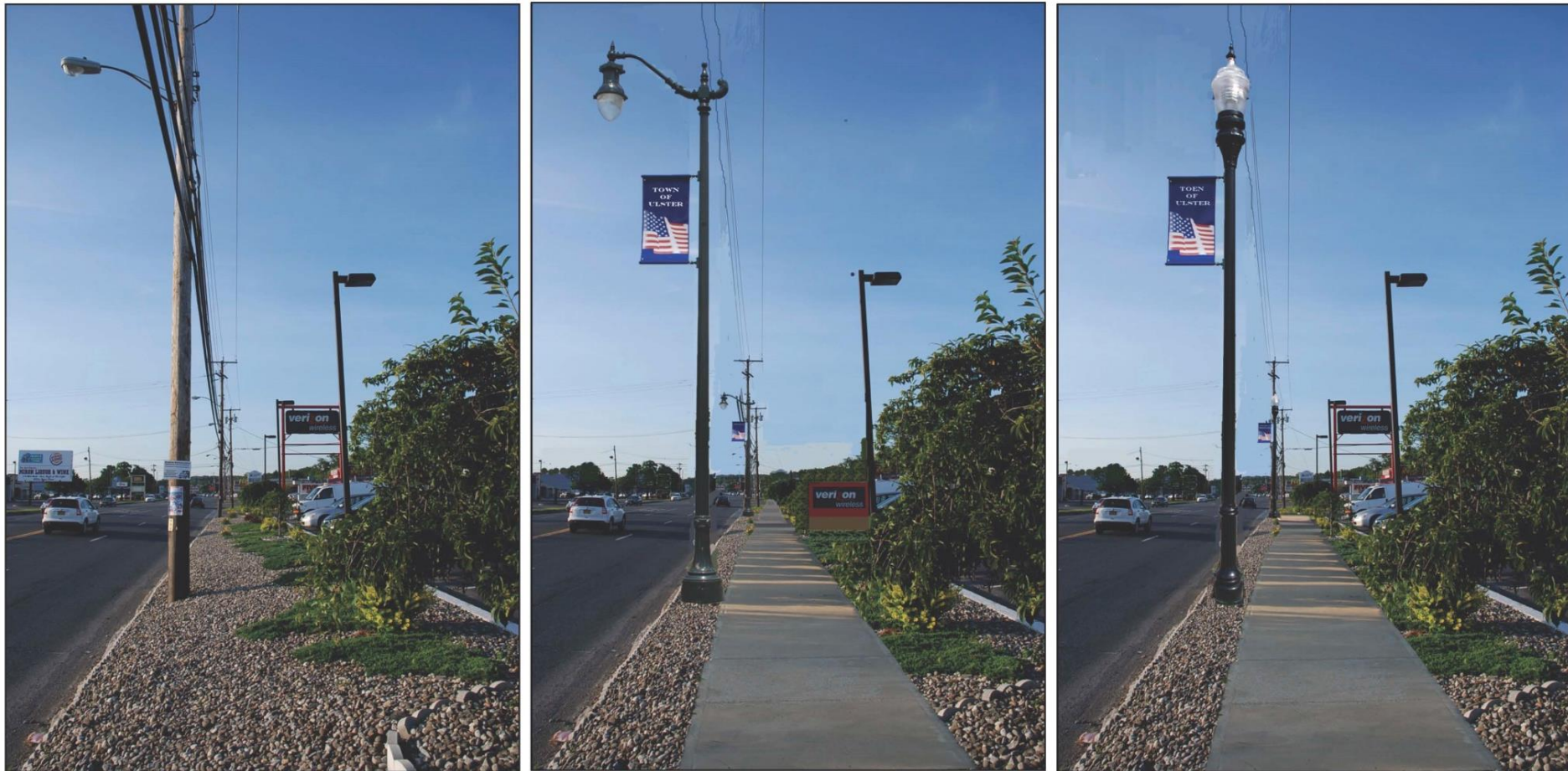
Above (Left to Right): View of existing conditions on U.S. Route 9W corridor looking north from Kings Mall on east side of U.S. Route 9W; same view showing new period streetlights with banners, a new sidewalk, relocation of telephone and cable lines (see Appendix A) replacement of Verizon pole sign with monument sign and removal of billboard and pole signs on left side of photo; and same view with new period lighting with banner with the Verizon pole sign, but billboard on left side of photo removed. These illustrations show how streetlights, sidewalks and sign regulation affect the appearance of the corridor.
